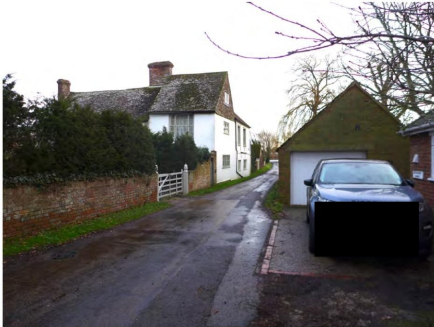
17. Manor House from N showing application site garage right.
