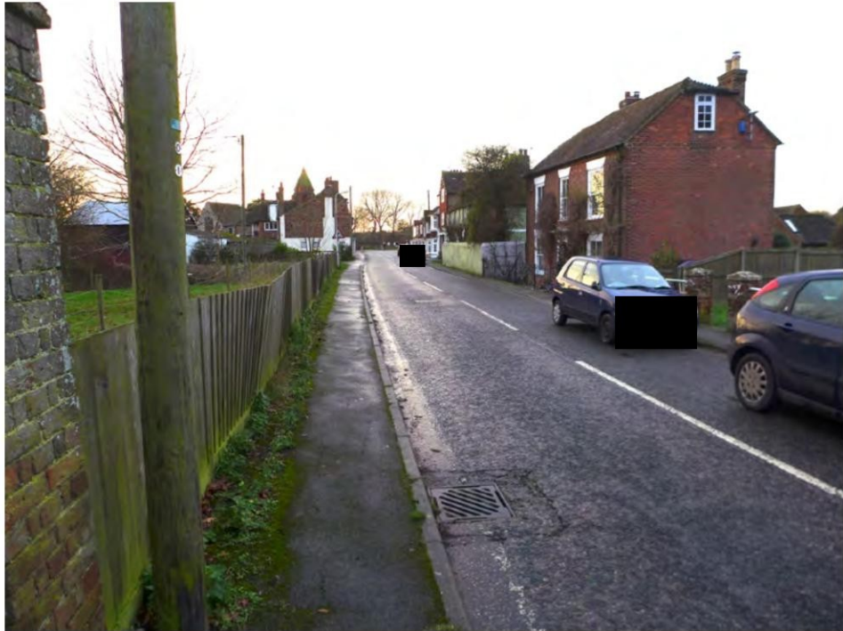
19. Pear Tree House from E, Brookland House beyond showing front boundary of application site left (wall proposed to replace fence).
