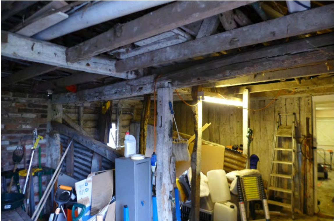
8. Interior of historic centre area looking S showing loft joists top and boarded partition adjoining S garage in background.
