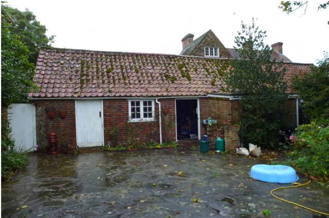
7. Outbuilding from W, Manor House beyond.
