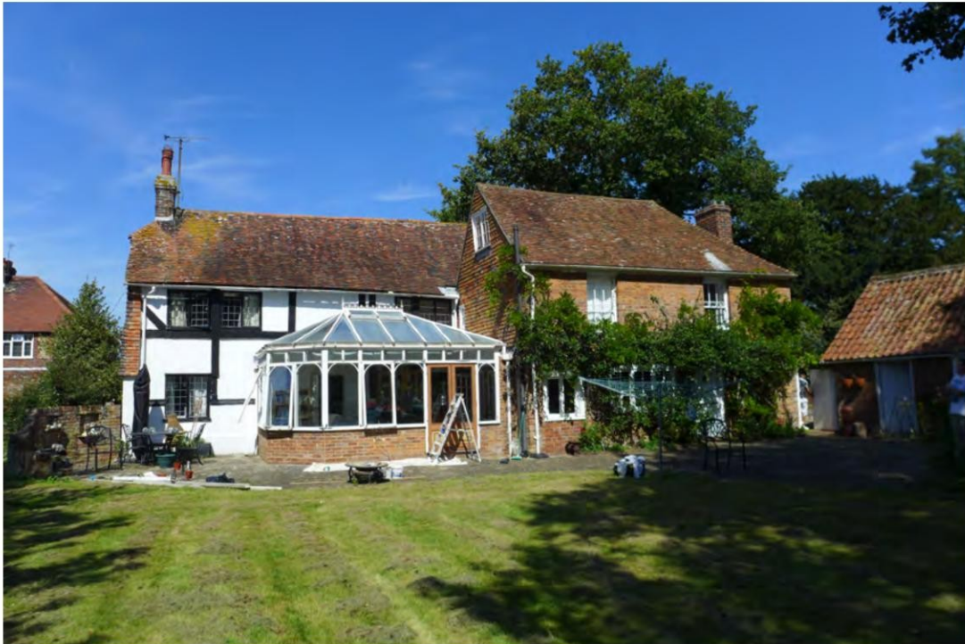
3. Rear of house (S), outbuilding right.
