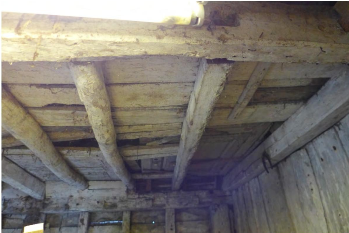
9. Historic centre area looking E showing studs and wallplate background, boarded partition right, loft joists and surviving floorboards top.
