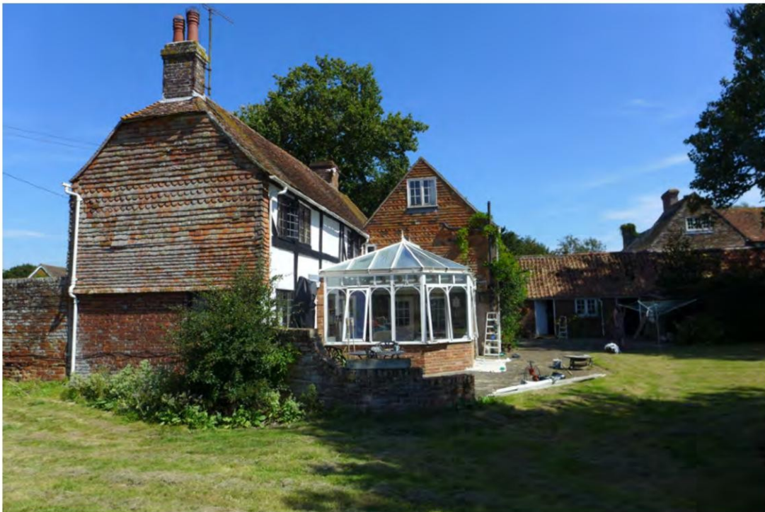
4. Side of house (W), outbuilding right, Manor House beyond.
