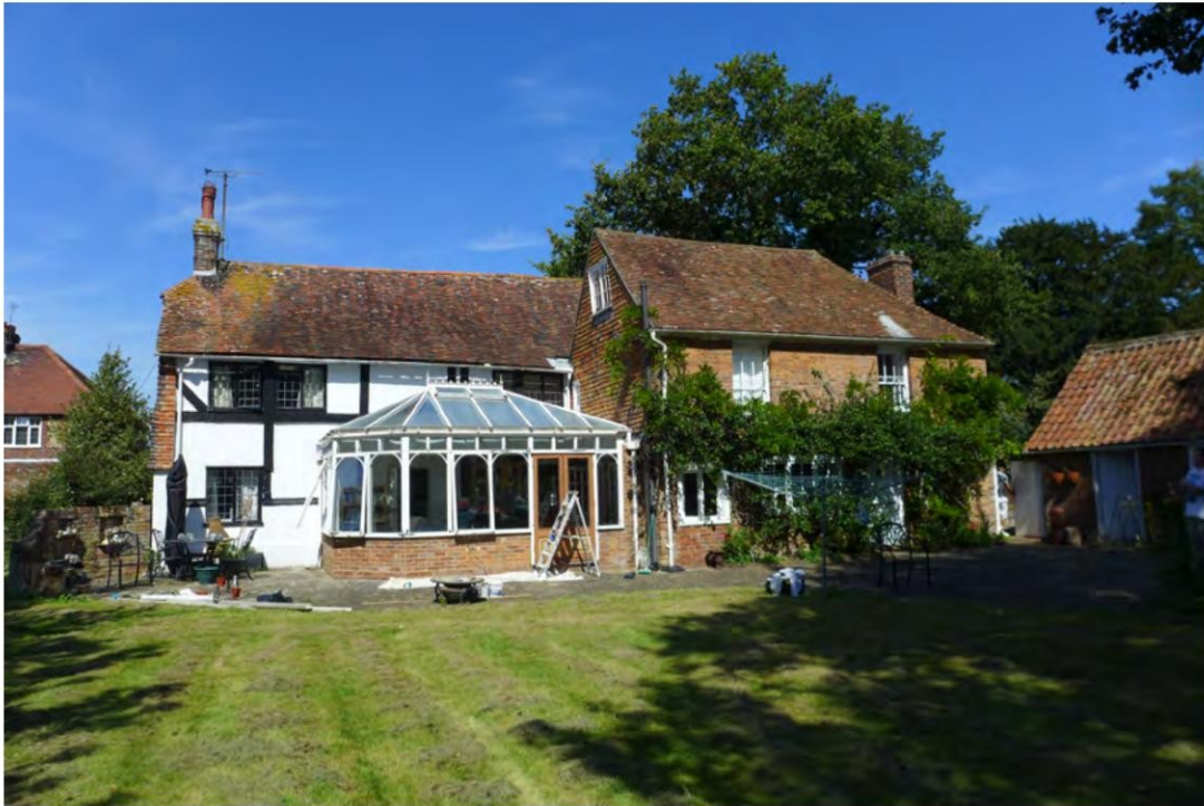
3. Rear of house (S), outbuilding right.
