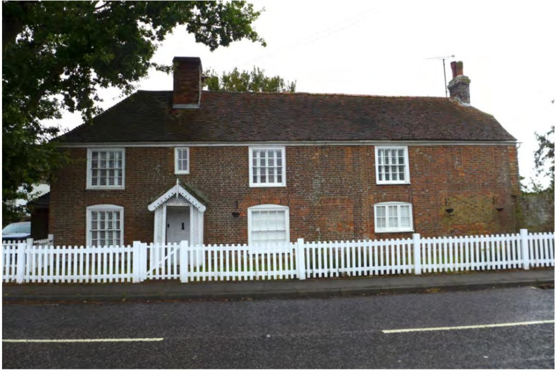
1. Front of house (N).
