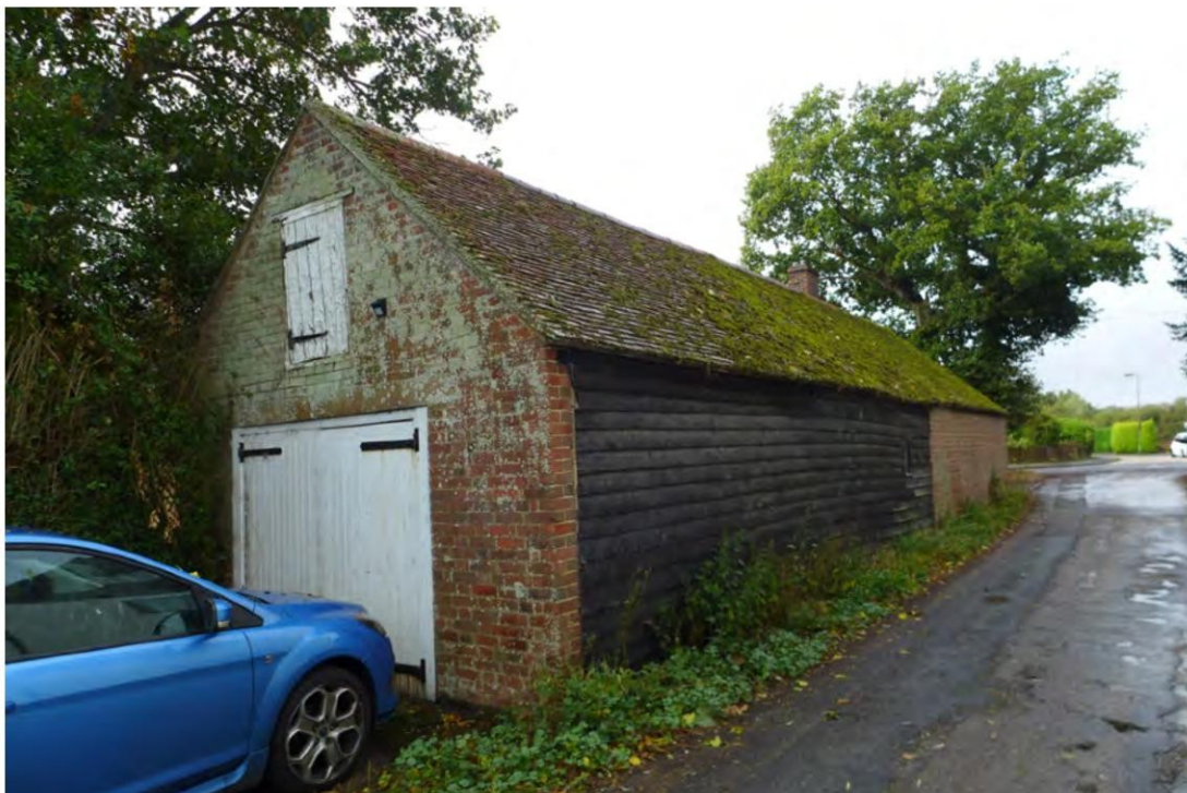
6. Outbuilding from S.
