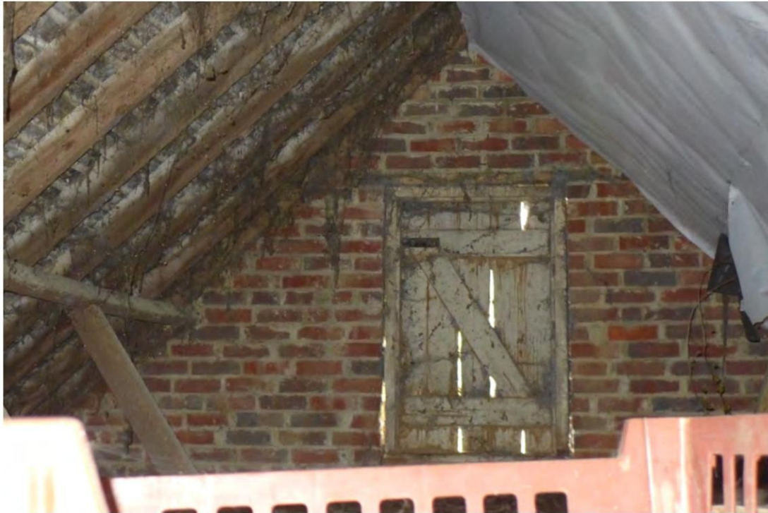
11. Roof space over S garage looking S showing loft external door and rebuilt roof structure.
