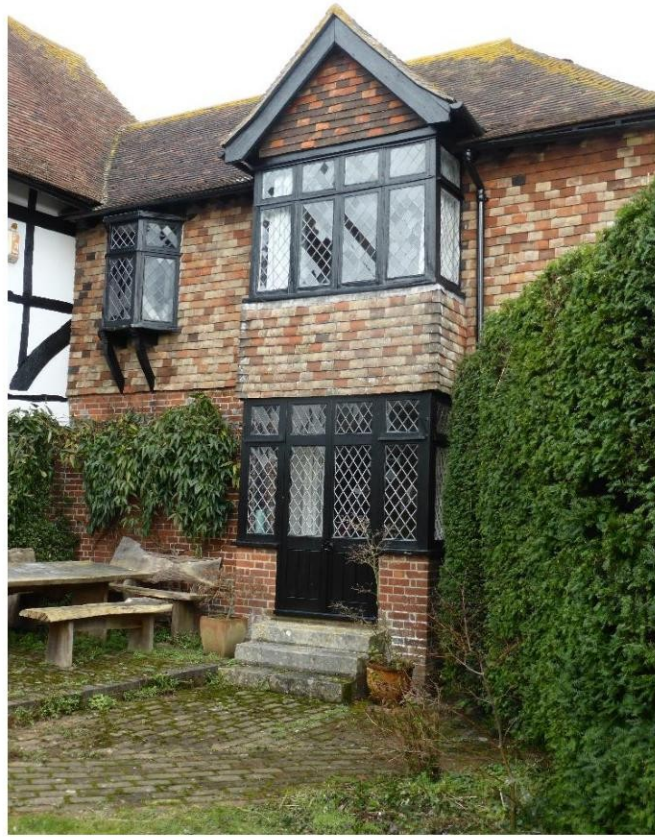
FIGURE 10 - BAY WINDOW SUBJECT OF REPAIRS
