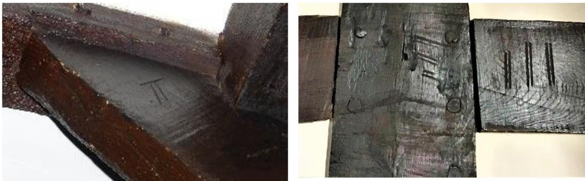
FIGURE 4 - EXAMPLES OF CARPENTERS MARKS
