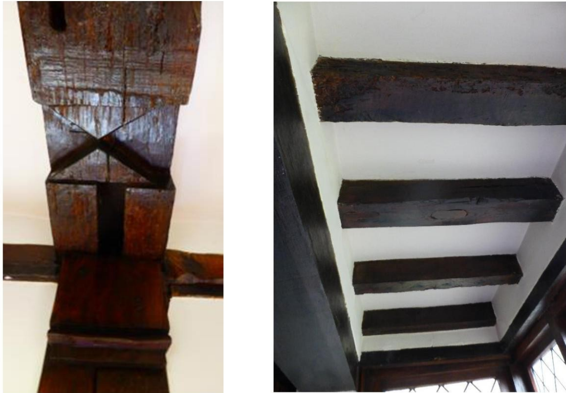
FIGURE 3 - DOUBLE DOVE TAIL JOINT AND REUSE OF TIMBERS IN BAY
