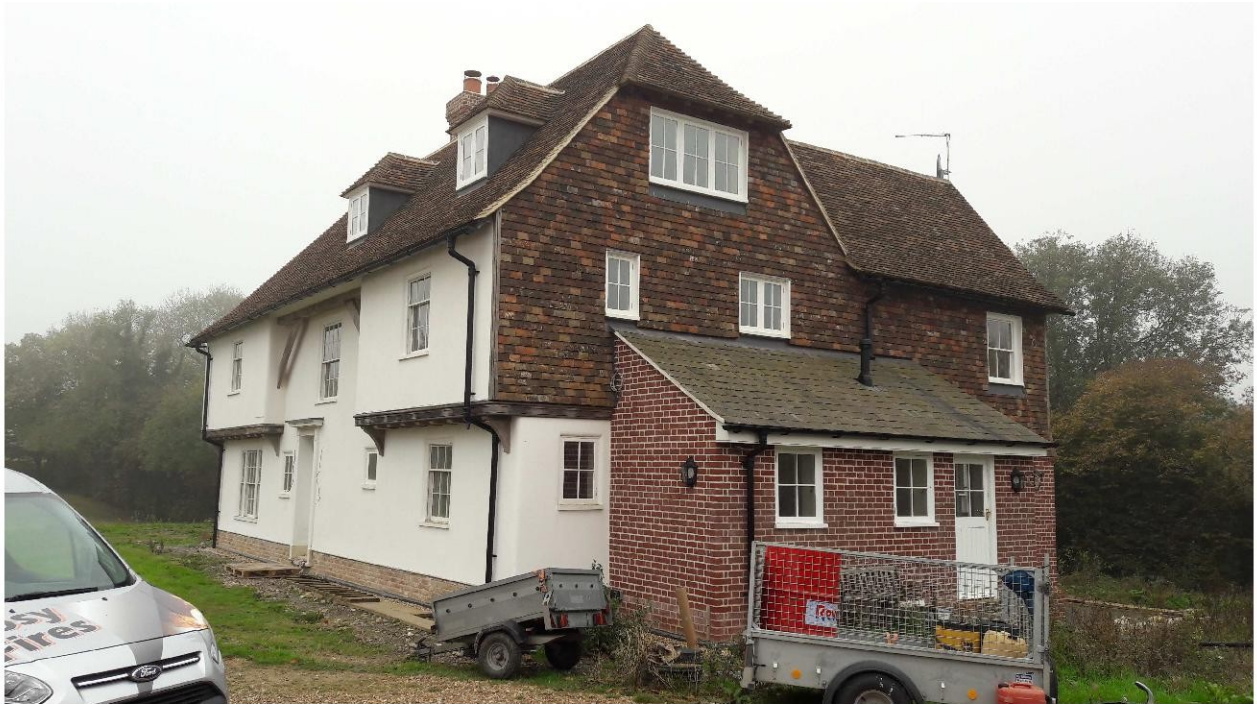
Fig 3 – Replacement dwelling from north nearing completion
