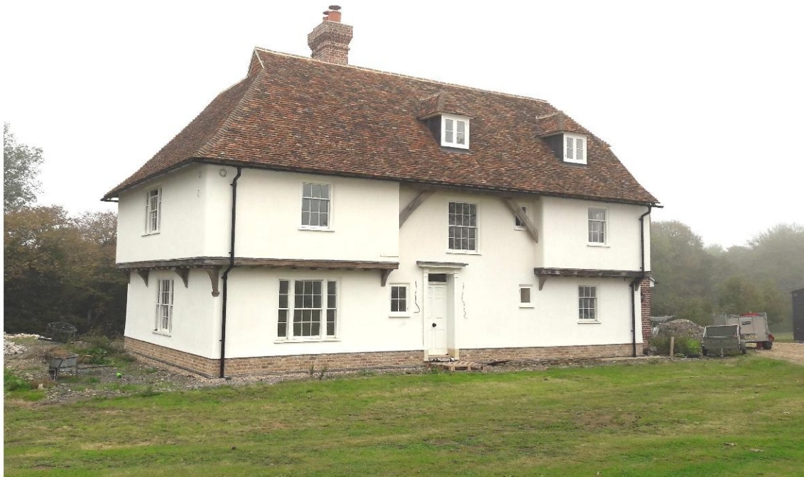
Fig 2 – Replacement dwelling from east nearing completion
