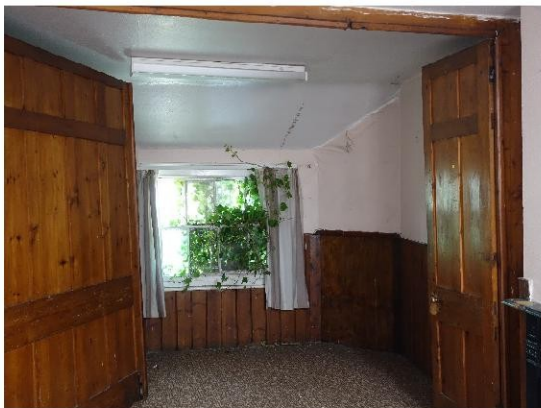
UPSTAIRS MEETING ROOM (TO BE BEDROOM)
