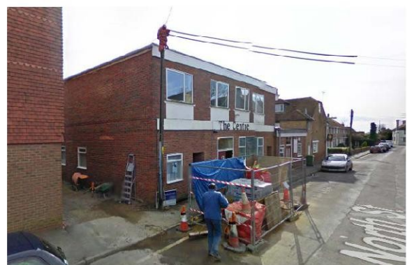
NEW COMMUNITY CENTRE OPPOSITE CHAPEL
