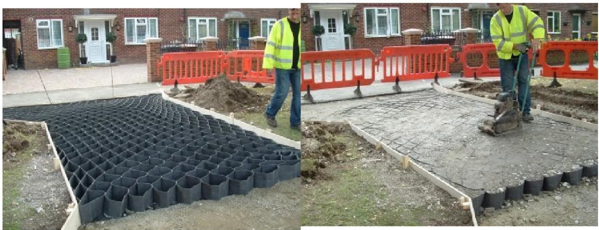
Figure 4: Photos, the courtesy of TERRAM Geosynthetics, showing the installation of a cellular confinement system.
