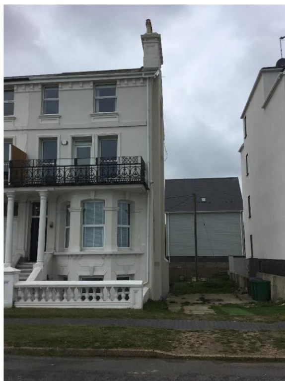
Front of property with. Photographer facing west.
