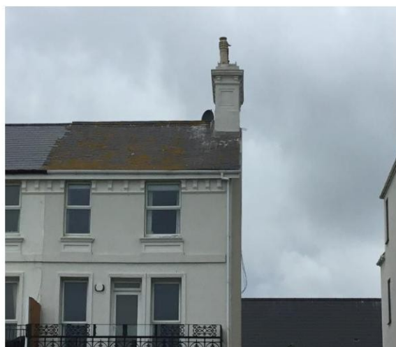
Front of property showing roof area. Photographer facing west.
