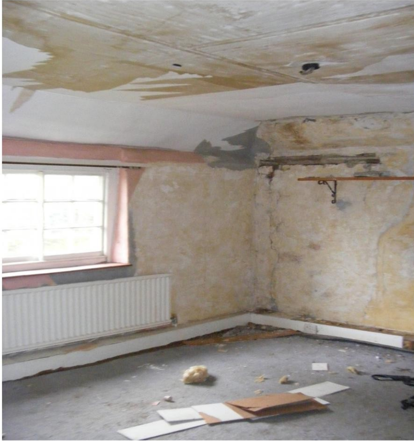
Bedroom 2 – Low Ceiling Height (to increase ceiling height to match Existing Bedroom 1)
