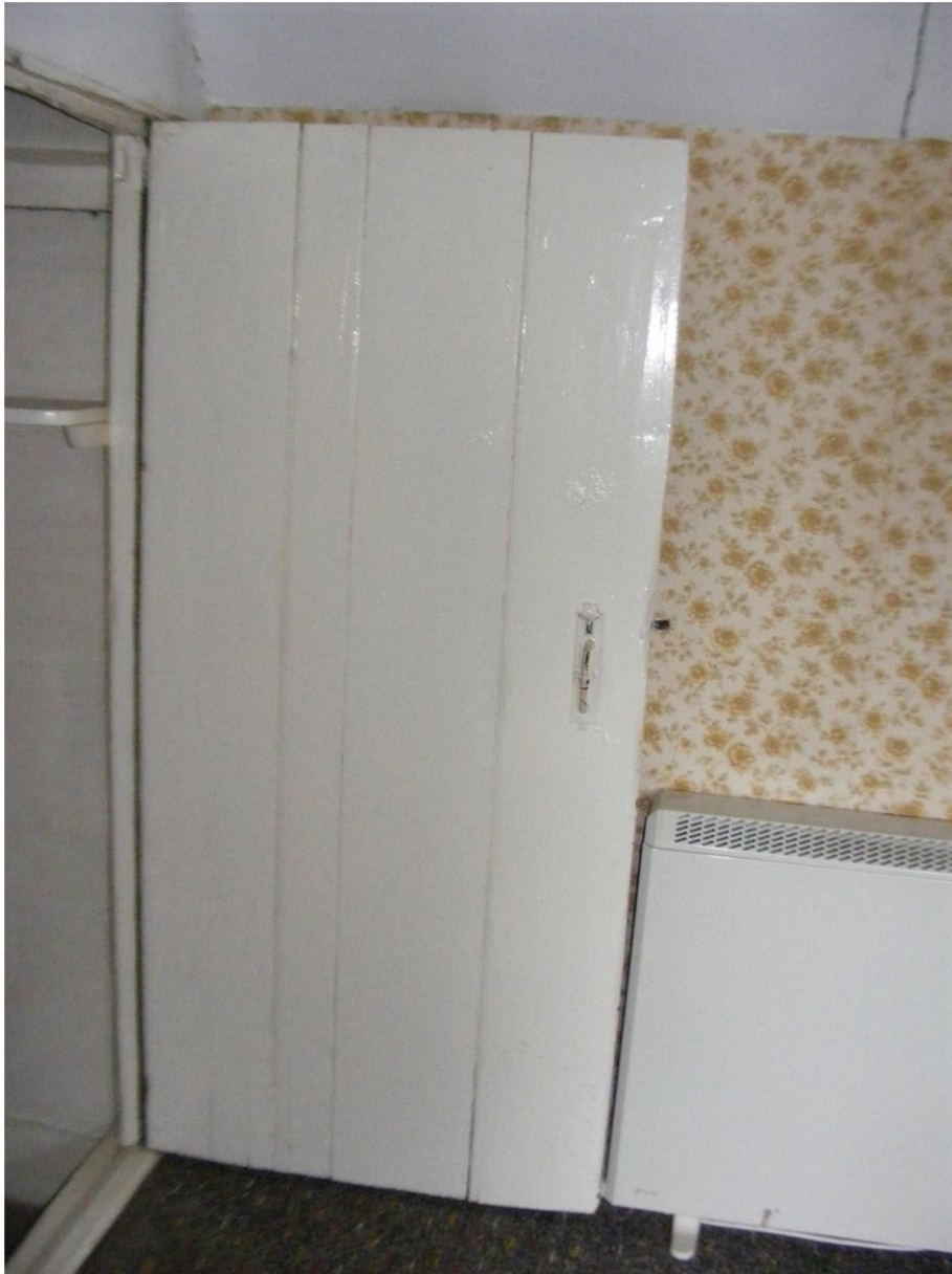
Existing Wide Boarded Ledged Plant Internal Door (To be retained)
