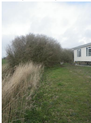
Figure 8: THE WESTERN DRAIN.
