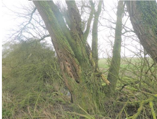
Figure 6: THE SOUTHERN DRAIN SHOWING THE BLACKTHORN SCRUB AND THE POTENTIAL BAT ROOST CRACK WILLOW.
