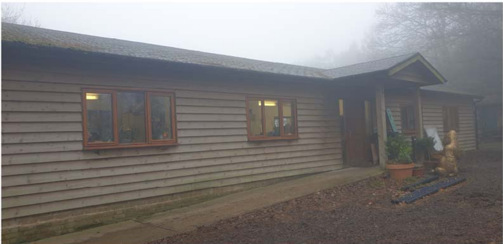
The northern elevation of building B1
