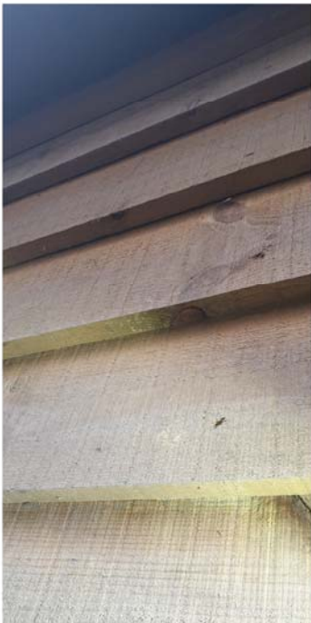
Weatherboards of building B1
