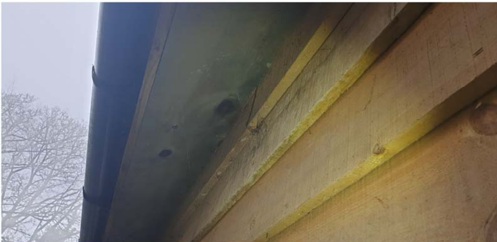
Eaves of building B1
