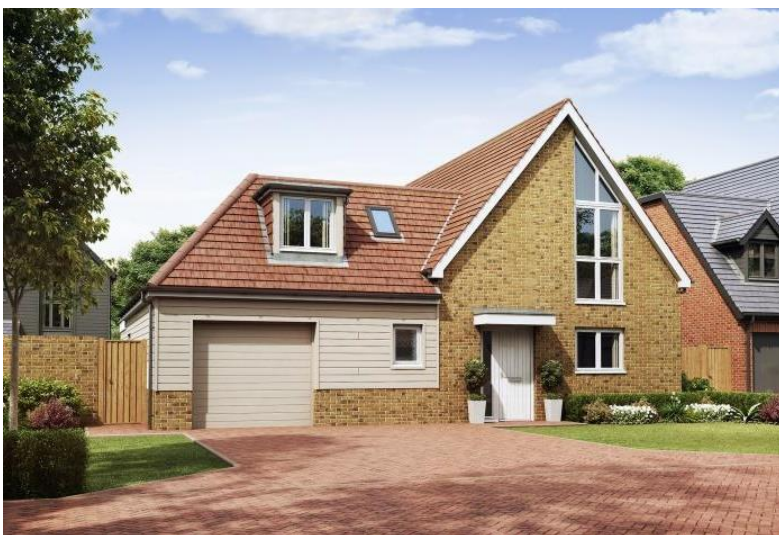
New builds to the east end of Cockreed Lane
