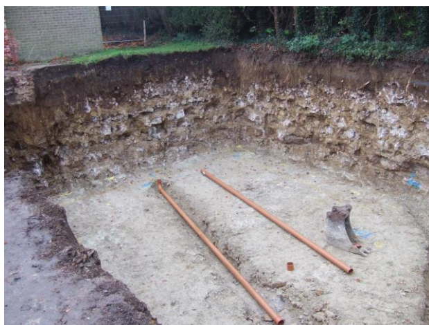
Basement level for the coach house rebuild 2018
