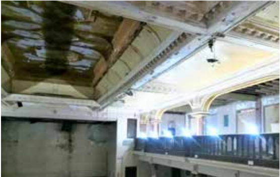
14. The highly decorative ceiling and lantern ceiling feature will be restored.
