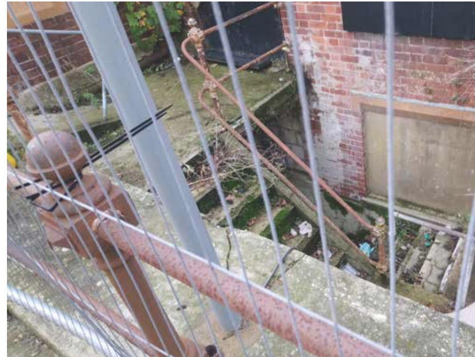
Photo 20: Side elevation from Longford Terrace car park
