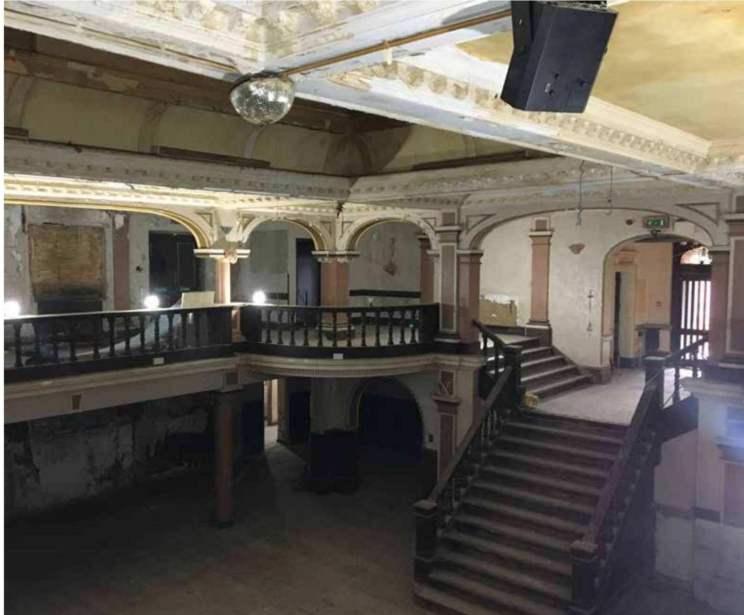
11. The Leas Pavilion has an ornate interior that will be carefully restored in line with heritage advice.
