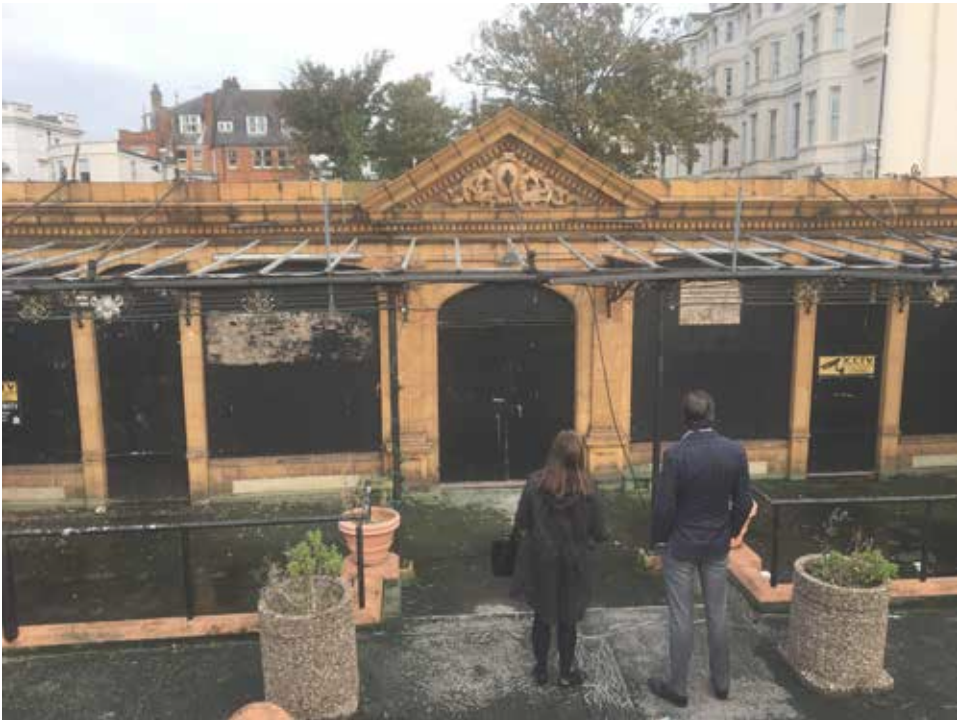
Photo 7: Front terracotta elevation
