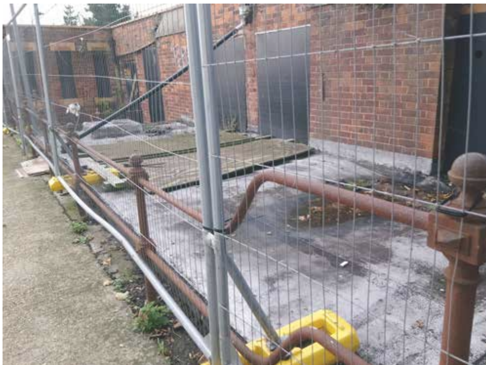
Photo 19: Side elevation from Longford Terrace car park
