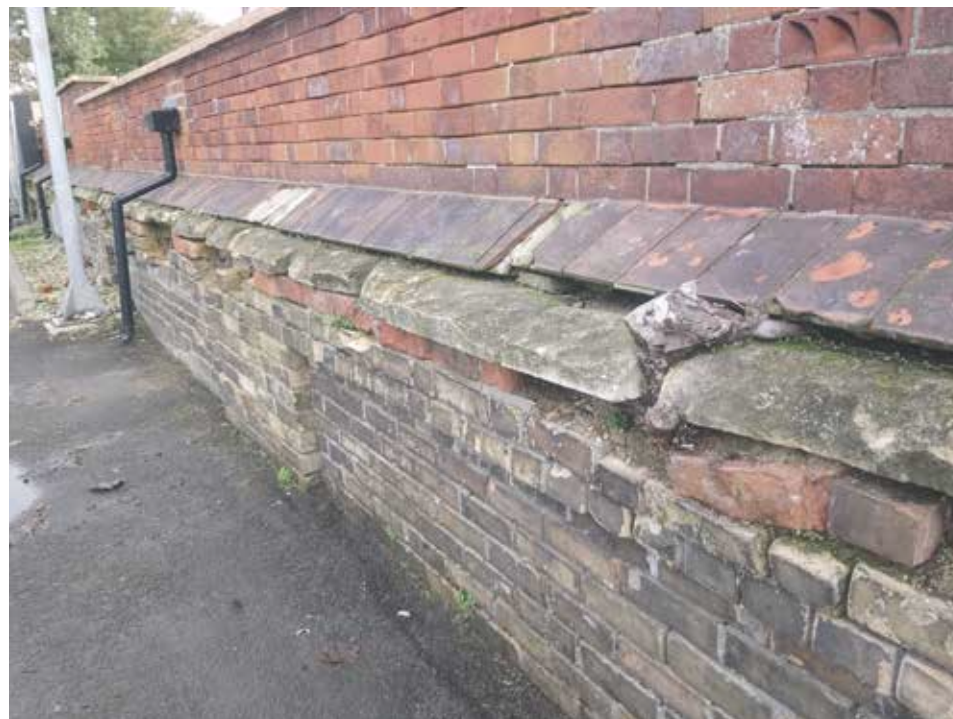
Photo 15: Masonry wall to Cheriton Place car park
