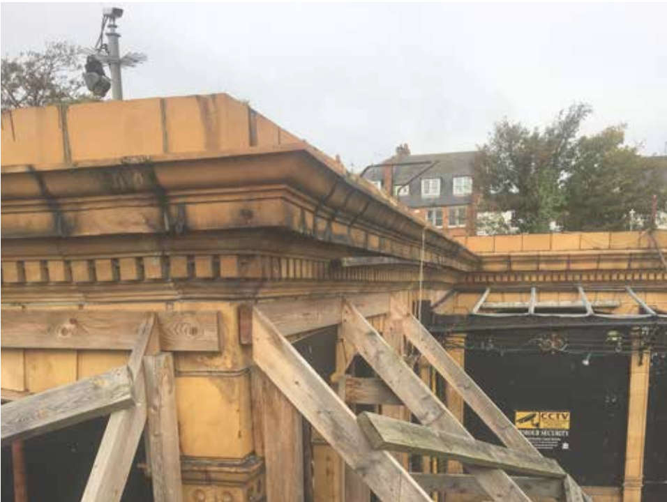
Photo 8: Cornice detail and temporary propping
