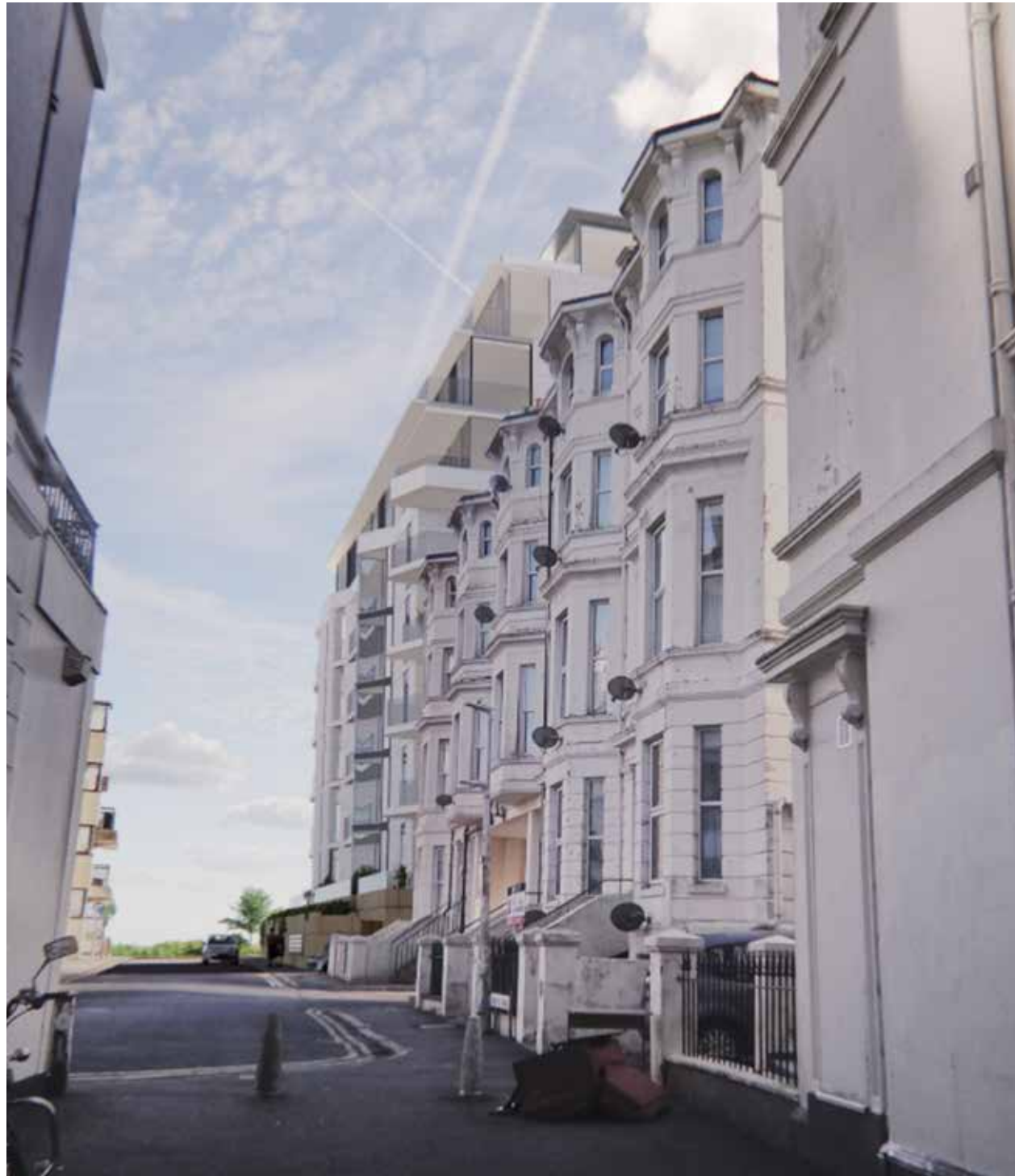
View along Longford Terrace
