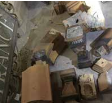
4. Broken terracotta pieces from the front facade have been salvaged and will be repaired and returned to their previous locations where possible.
