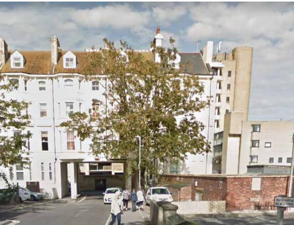
Photo 4: View of Longford Terrace
