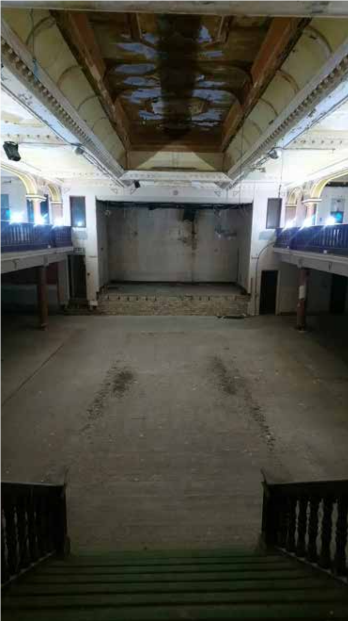
6. The stage has been stripped to a bare concrete structure which dominates the interior of the main hall.
