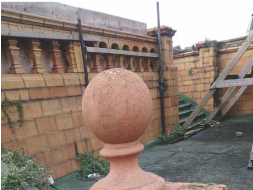
Photo 10: Detail of front courtyard wall
