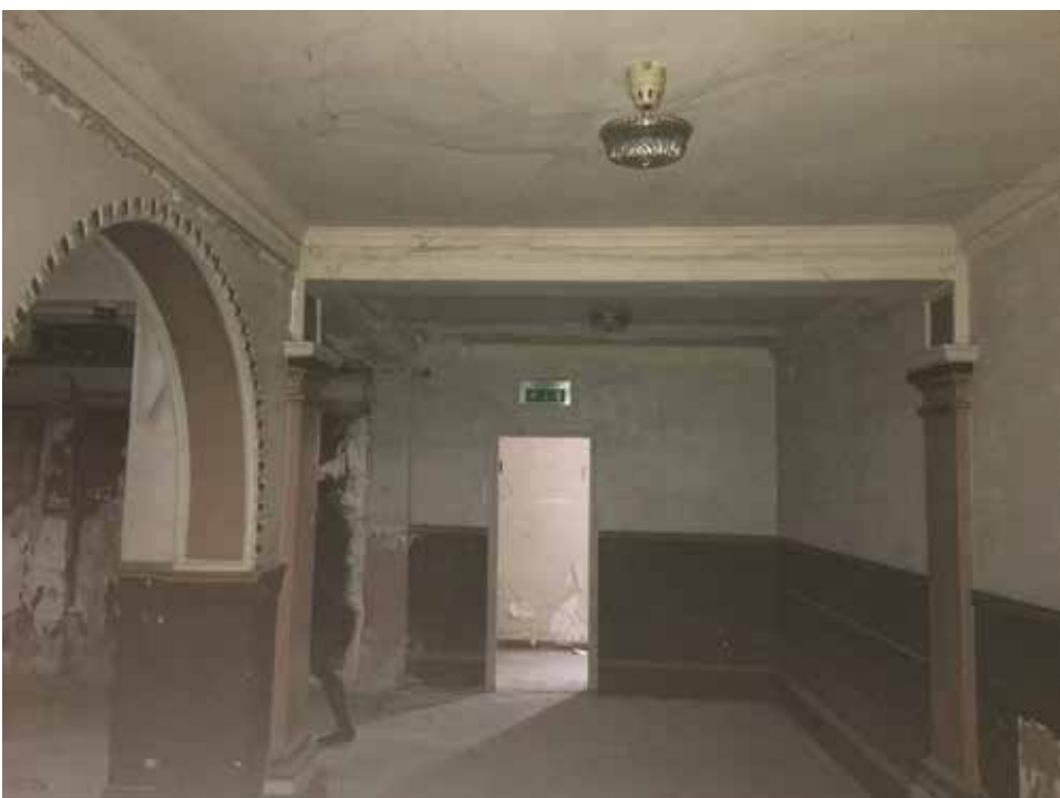
Photo 25: Beneath the NE gallery
