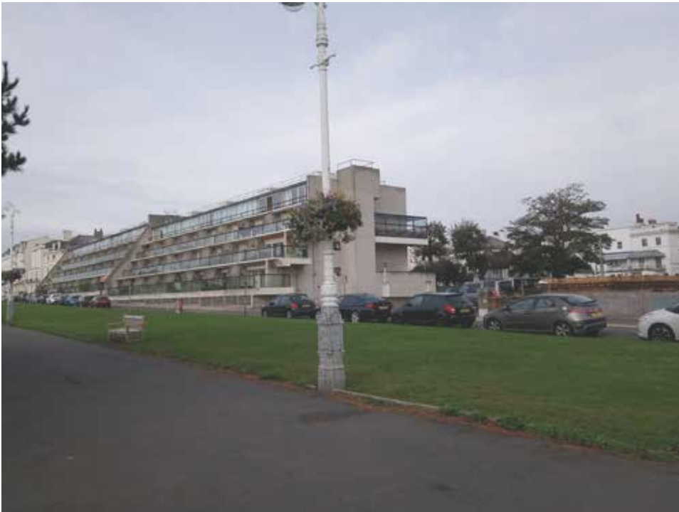
Photo 2: Site and its surroundings SW side (Apartment block, White Cliffs)
