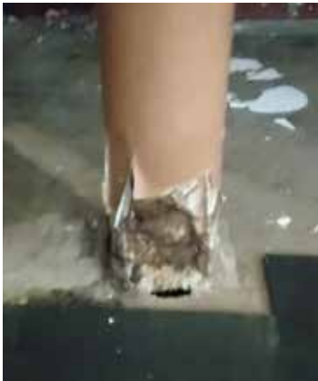
9. The columns in the main auditorium will be restored.
