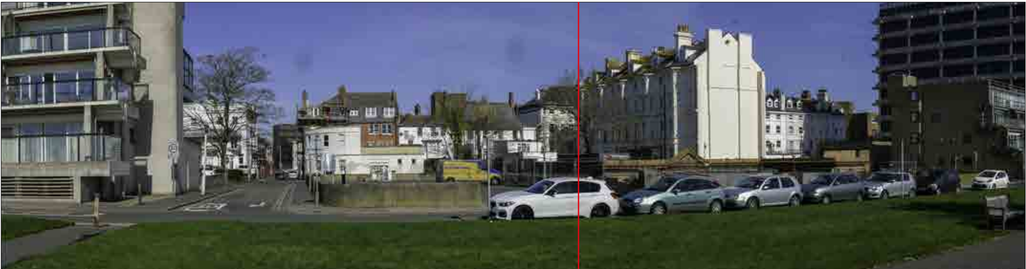
Approximate centre of site
