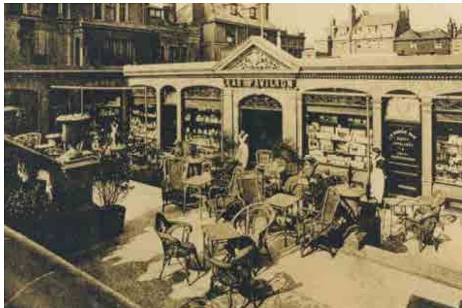
Fig. 36: Photograph taken from the pavement looking down at the frontage, tables, chairs and shops in the courtyard (reproduced from https://www.leaspavilionarchive.org.uk/ , from the private collection of Alan Taylor).
