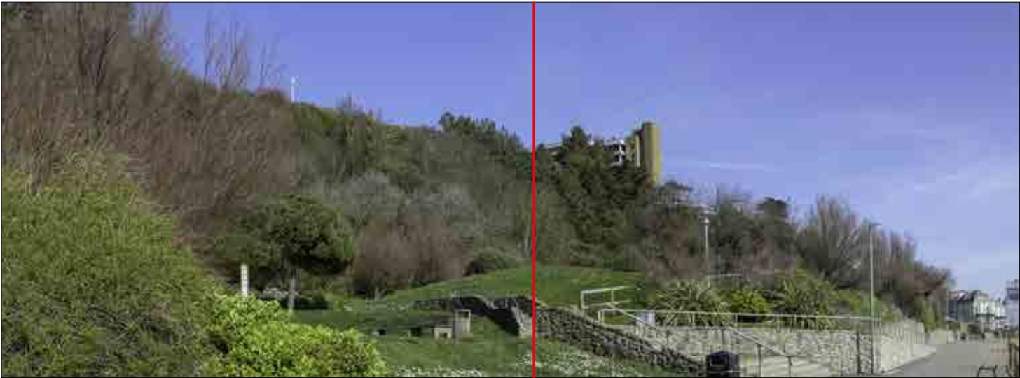
Approximate centre of site
