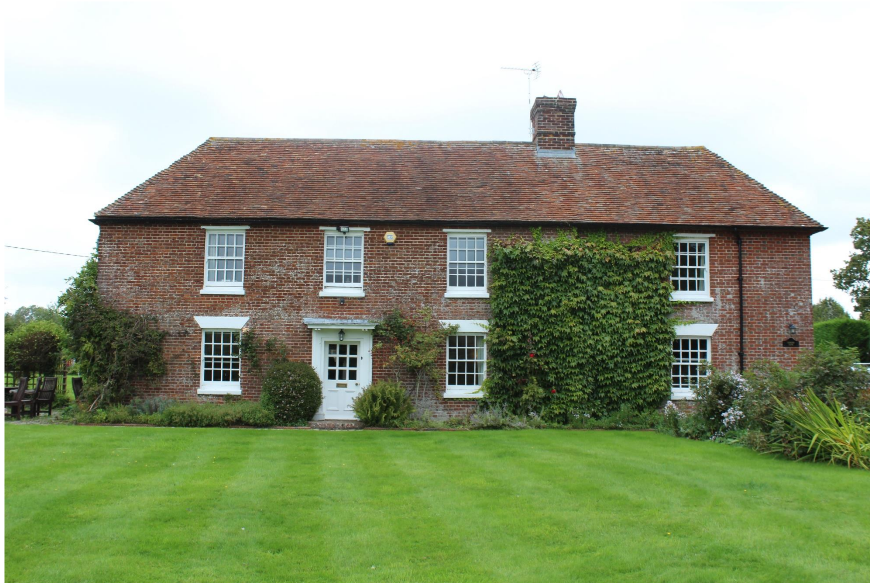
Front (south west) façade of Thornby Farm
