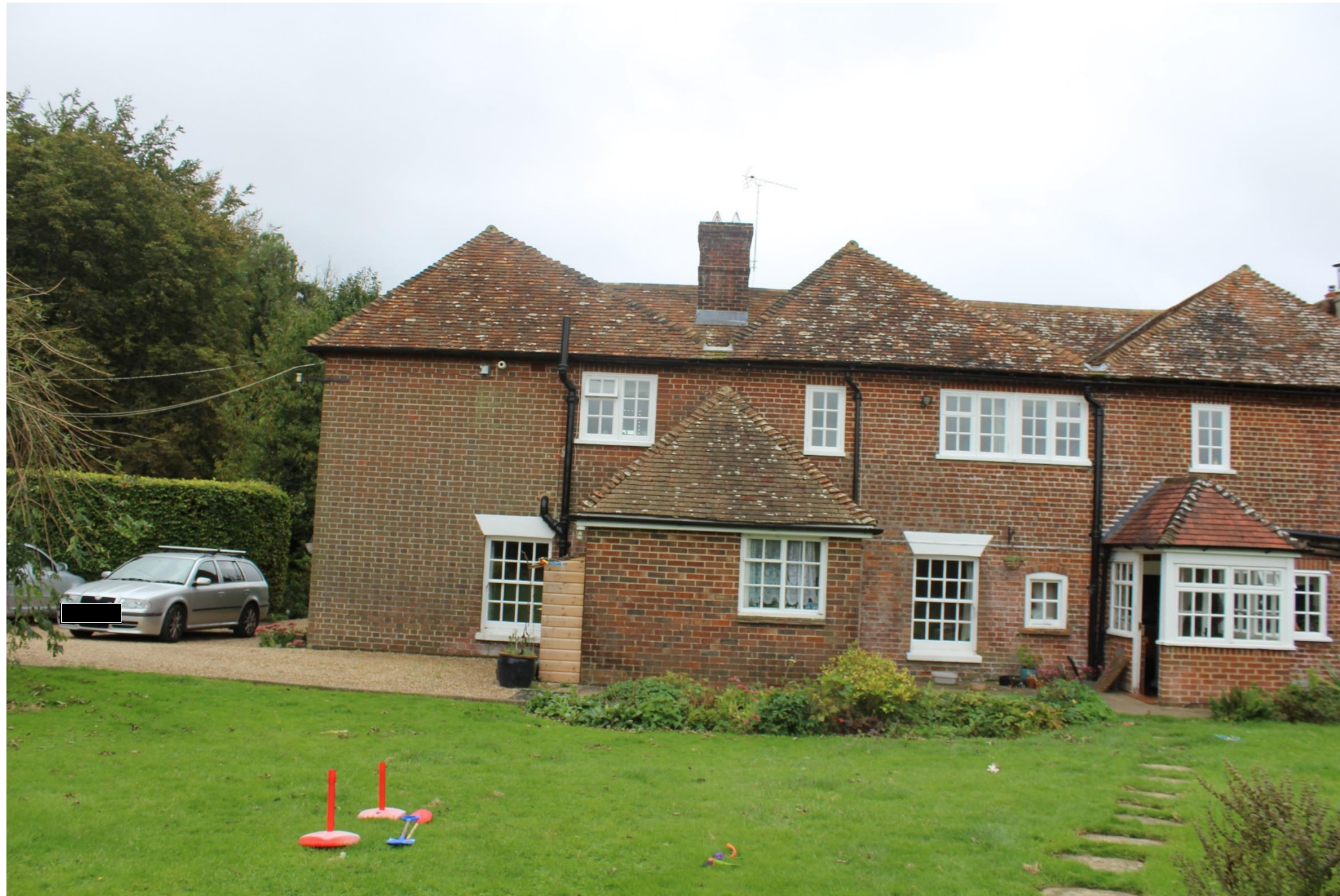
Rear (north east) façade of Thornby Farm showing the two single storey extensions to be demolished
