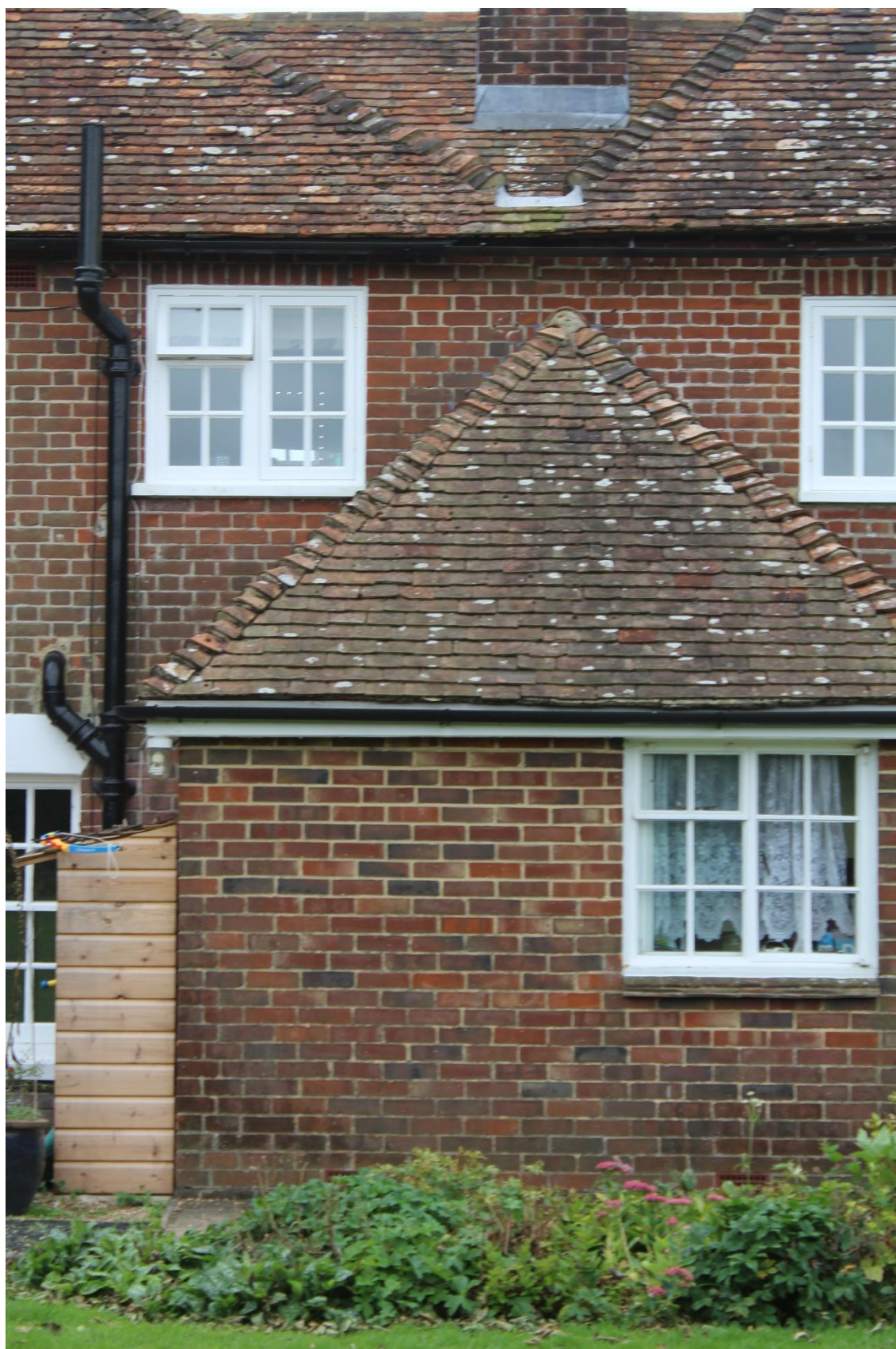
Existing rear extension
