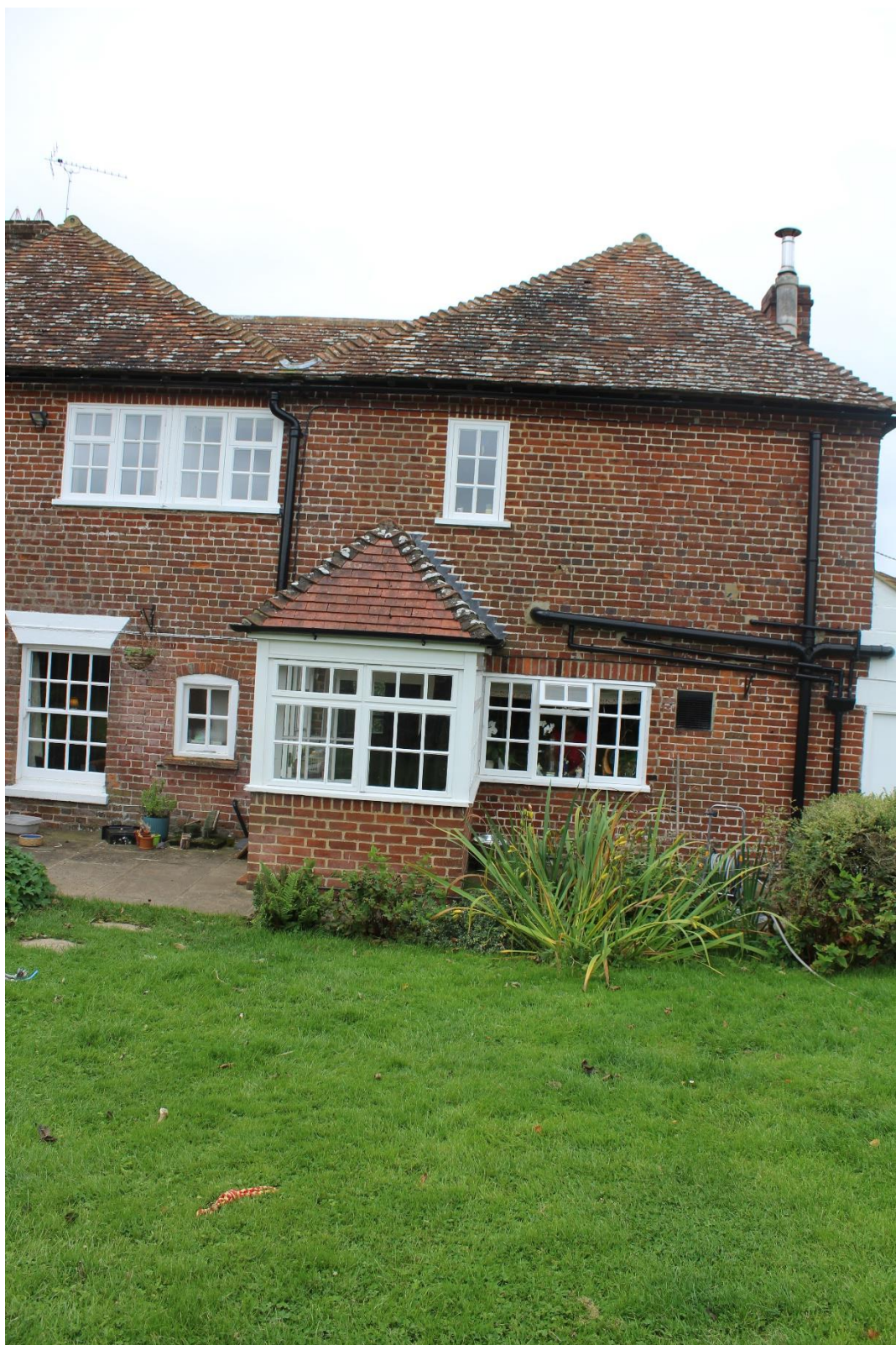
Existing rear extension
