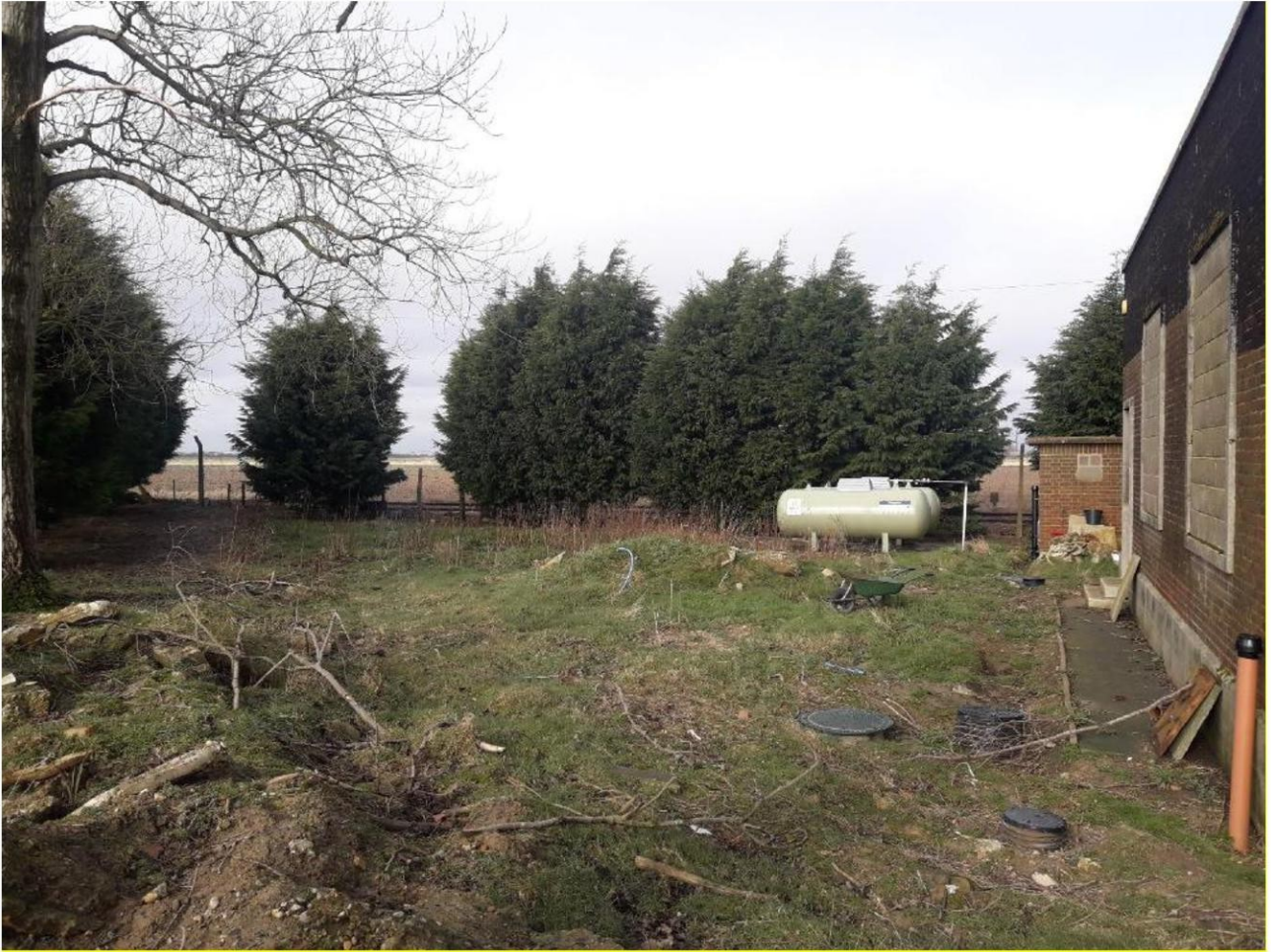
Plate 8: Proposed private garden area with visible services including septic tank. Railway track visible adjacent, propane gas tanks and additional rubble piles.
