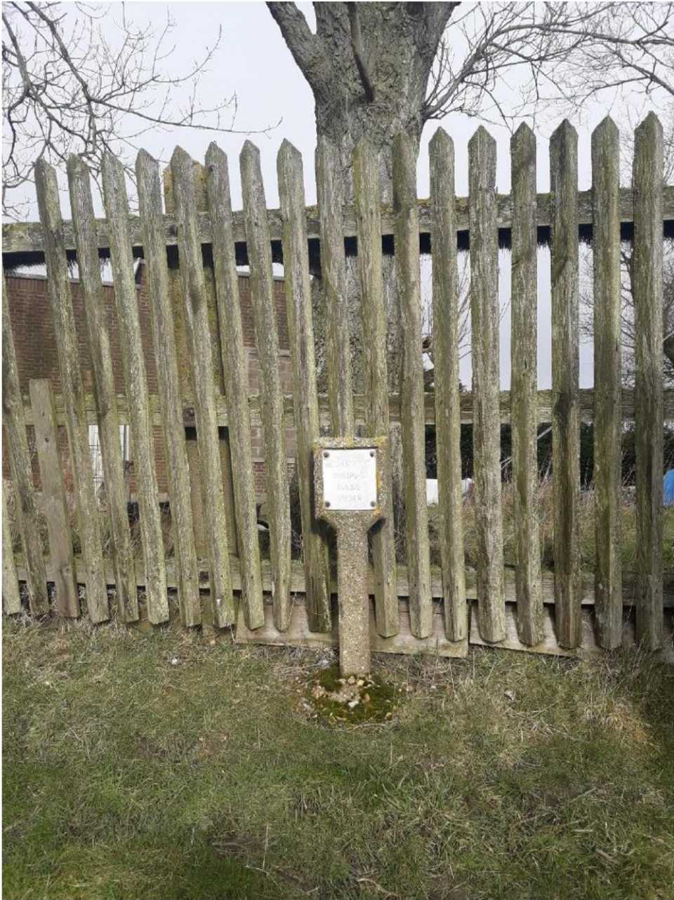
Plate 12: Water pumping mains marked near discharge point into drainage channel
