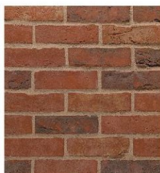
⑤ Red multistock brickwork with natural colour pointing
