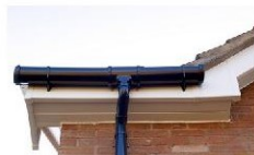
③ Upvc White Fascia and soffits. Black plastic gutters and downpipes
