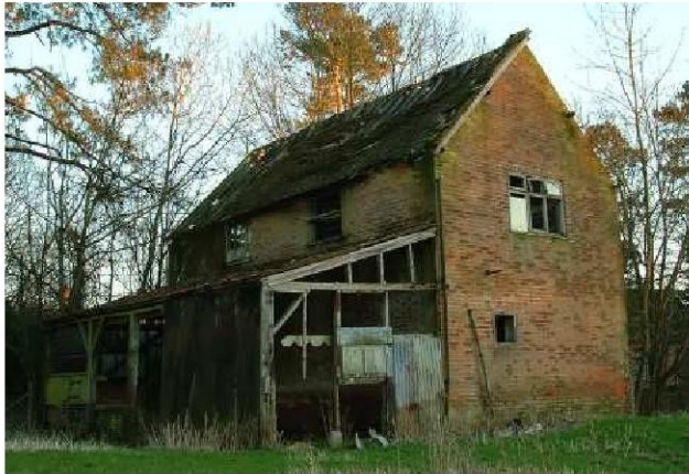
Showing original granary, with adjoining timber outbuilding
