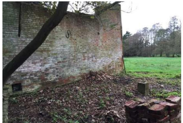
Rear view where timber framed structure used to sit
