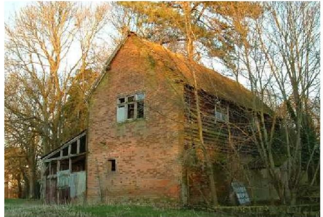
Showing timber cladding to granary's south elevation
