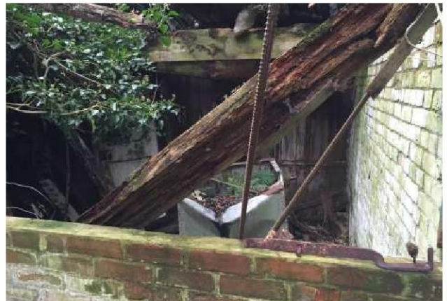
Debris resulting from collapsed roof
