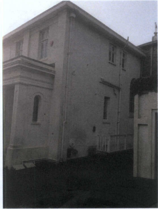
Fig 6 - Main house north elevation
