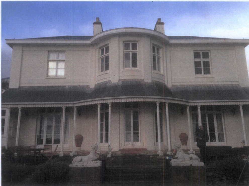
Fig 1 - Main house south elevation
