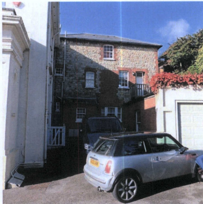
Fig 7 - East elevation of the annex
