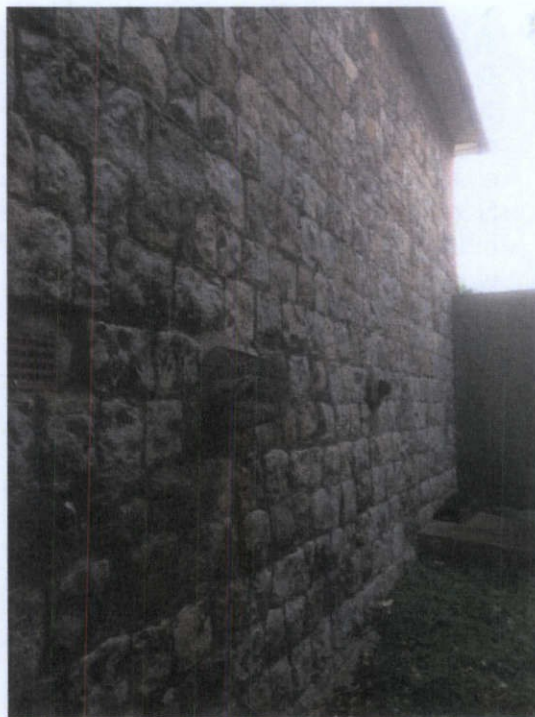
Fig 9 - North wall of ancillary block
