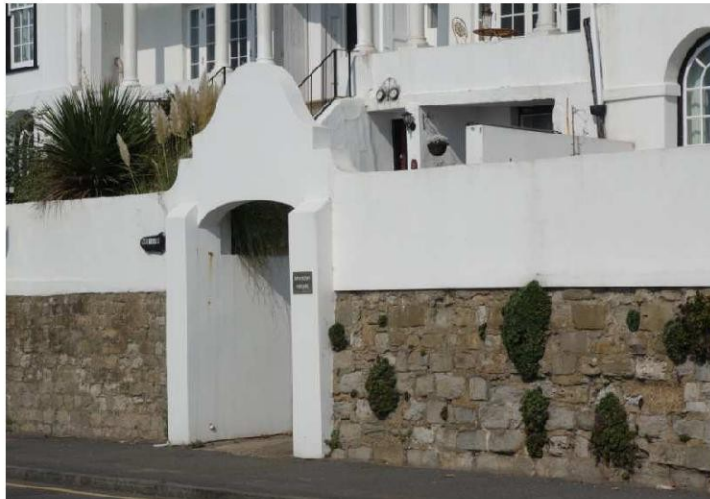
Adjacent wall type on Sandgate Esplanade
