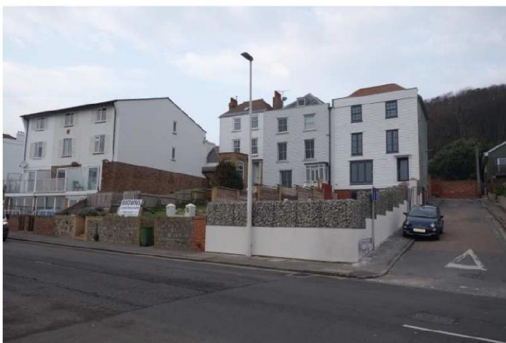
Wall at 32 Sandgate Esplanade
