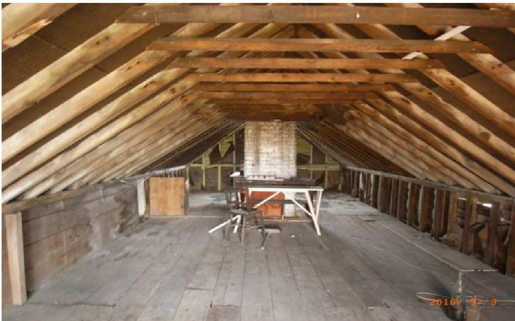
8. Internal view of loft space.
