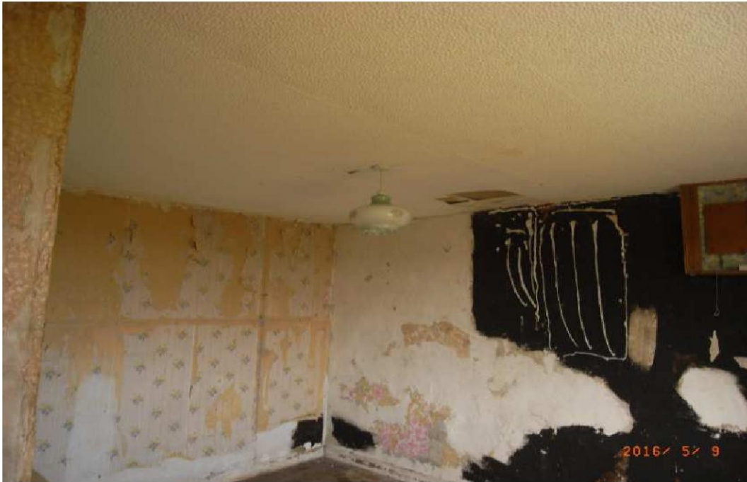
7. Internal view at ground level.
