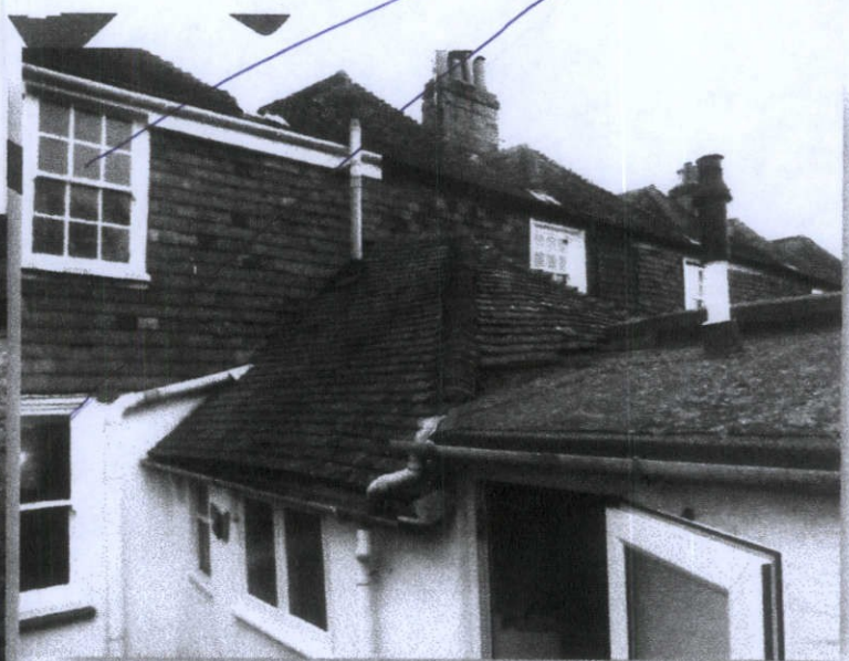
Hipped Roof over Kitchen meeting Flat roof over bathroom.
