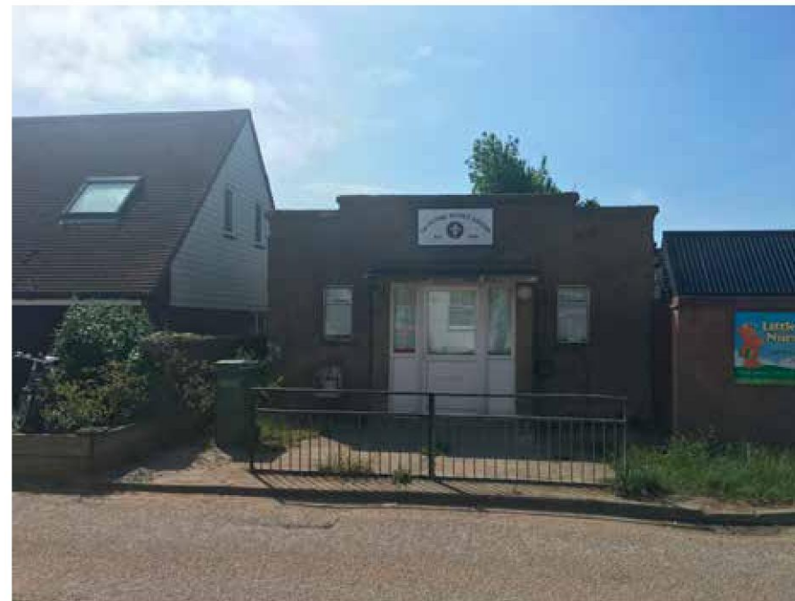
IMAGE D - Facing south towards existing Scout hut
