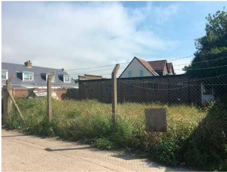
IMAGE C - View from access road on the west side of existing Scout hut
