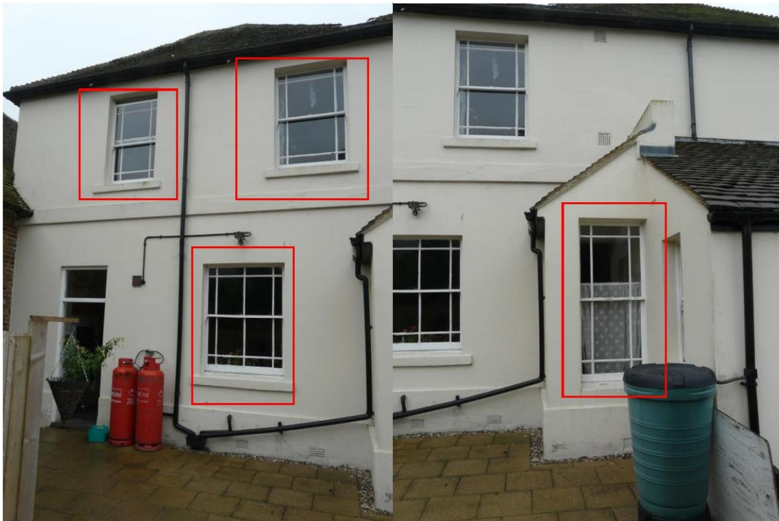
Photo 3. Rear side of the property. Proposed windows to be replaced.
