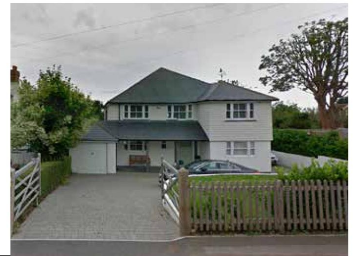
View of 2 storey residential property on Seabrook Road
