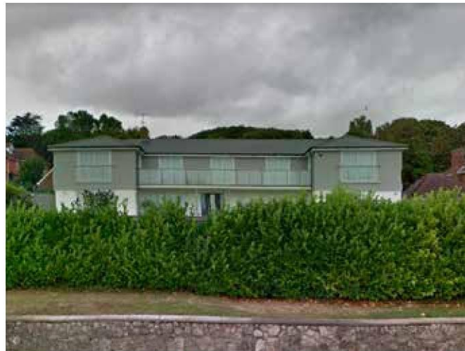
View of 2 storey residential property on Seabrook Road
