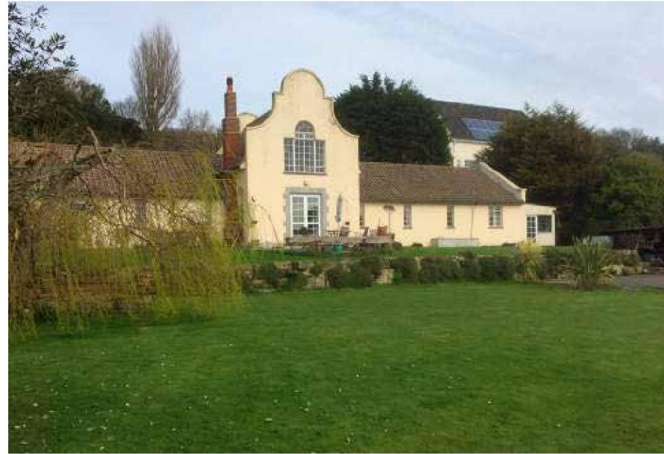
IMAGE B - View looking North towards the front elevation of the existing building
