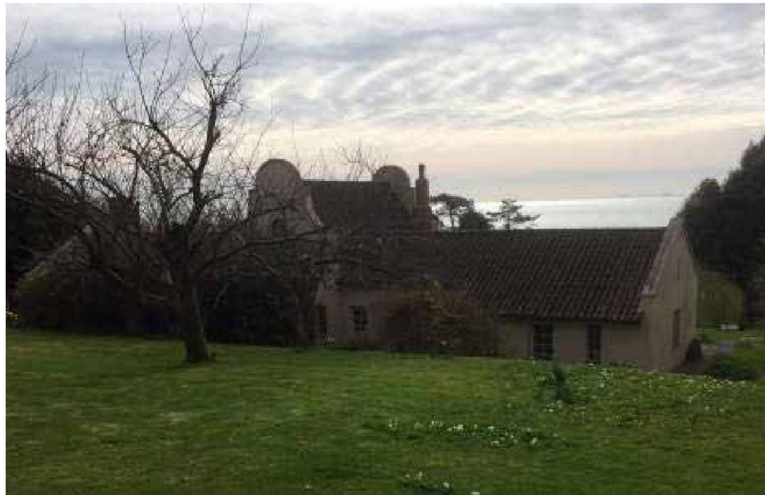
IMAGE C - View looking South East towards rear elevation of the existing building
