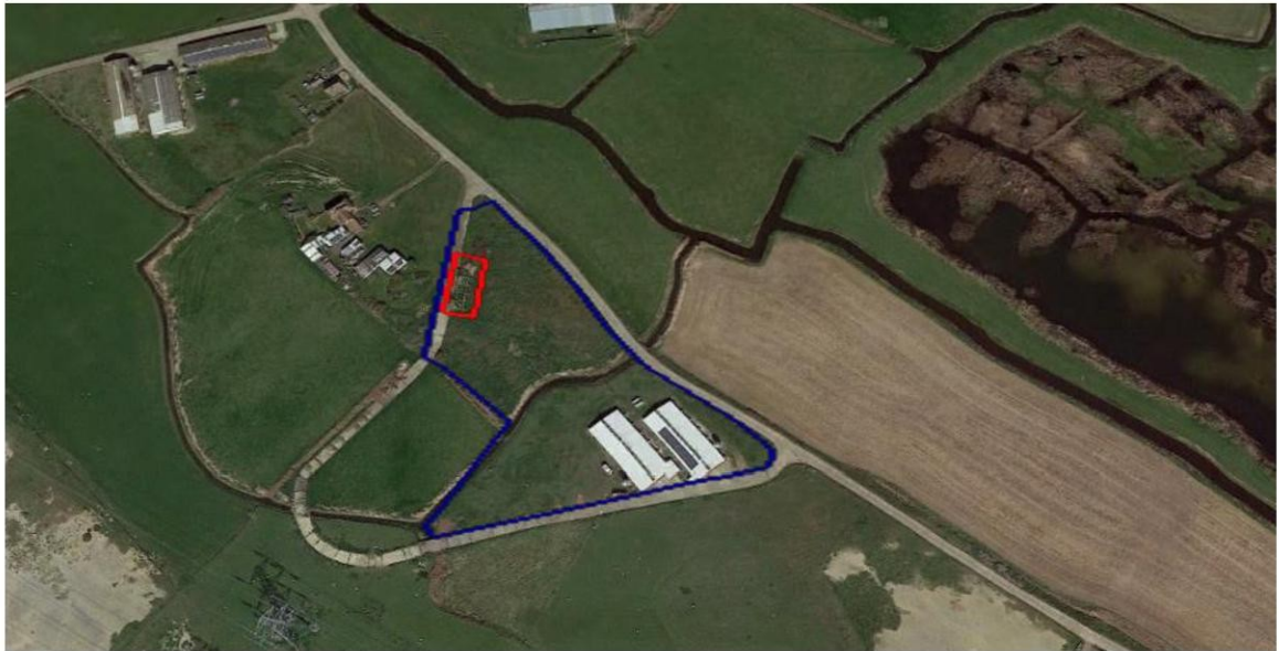
Fig. 1 Aerial view of the application site and Shinglebank Farm (Courtesy of Google Earth 2017)
