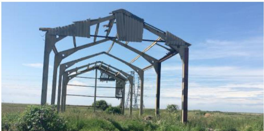
Fig. 4 Existing structure on the site
