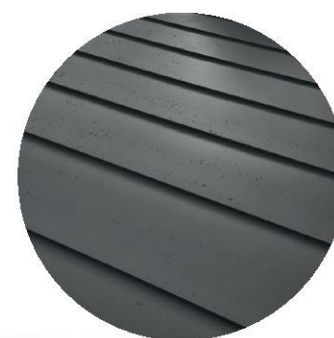
Standing Seam Zinc Roof
