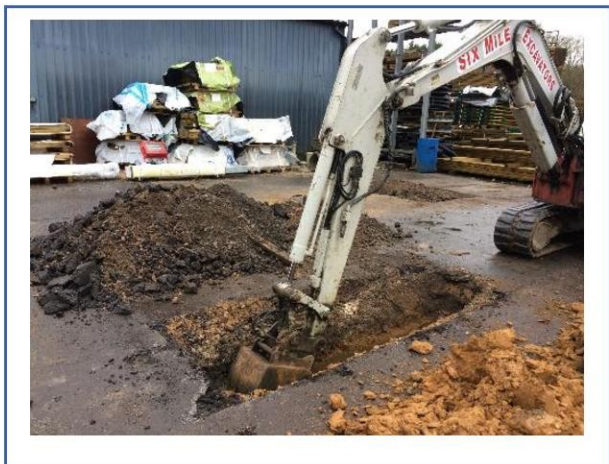
Trial pitting on site
