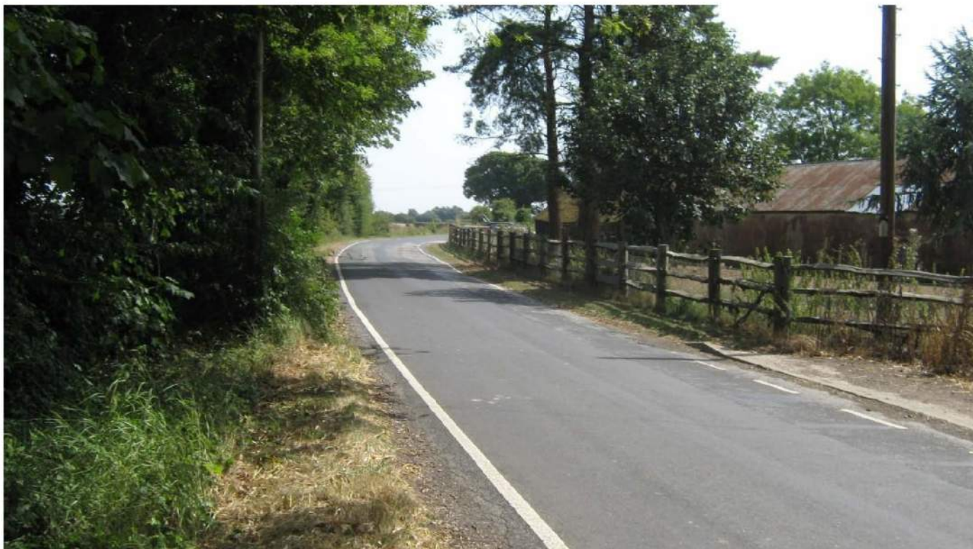
Photo 5 Visibility splay to the right of the existing access to be improved by setting back the length of fence shown in the photo.
