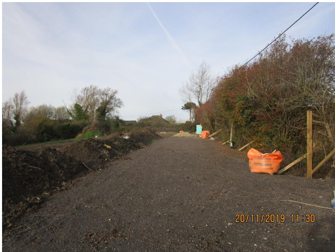
Photo 2 – View of the temporary access road looking north
