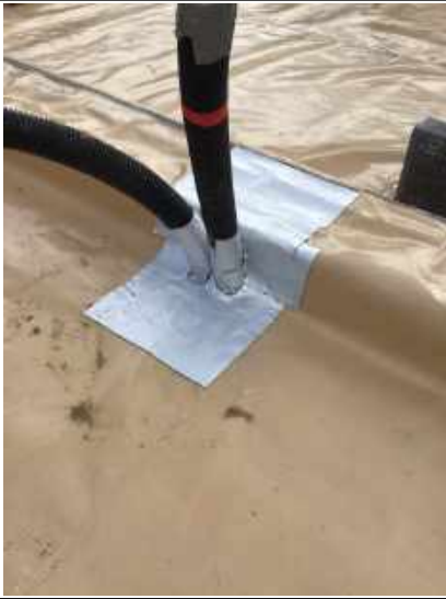
Another completed pipe penetration
