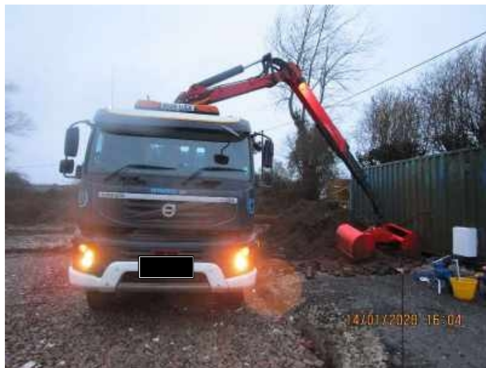
Photo 5 – Removal of asbestos impacted arisings via grab lorries
