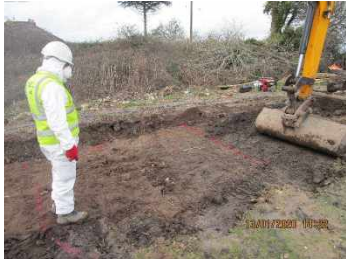
Photo 1 – Conduct of near surface remedial excavation under SEC Watching Brief
