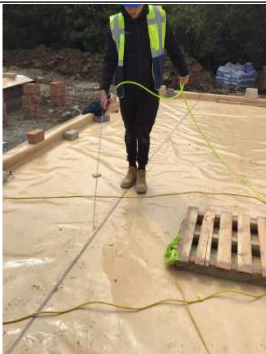
Air lance test carried out to a welded joint.
