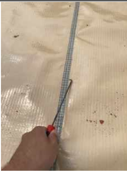
Pick and probe test to a welded lap joint in the membrane.
