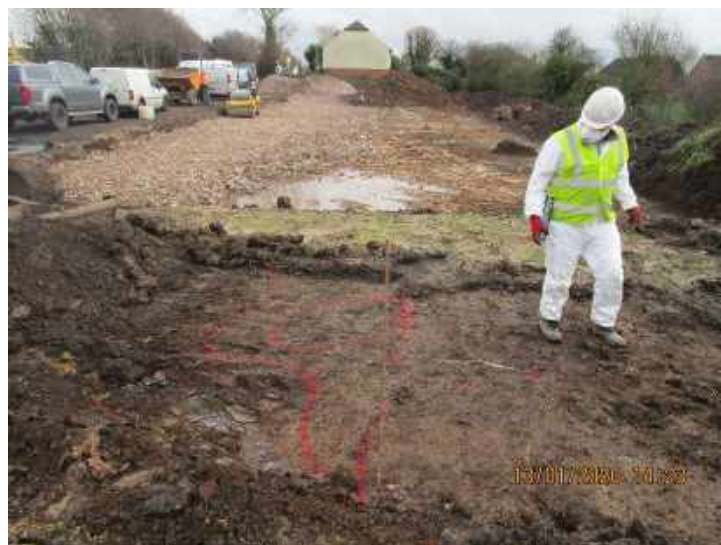
Photo 6 – Placement of imported crush pile mat material in the background beneath proposed houses
