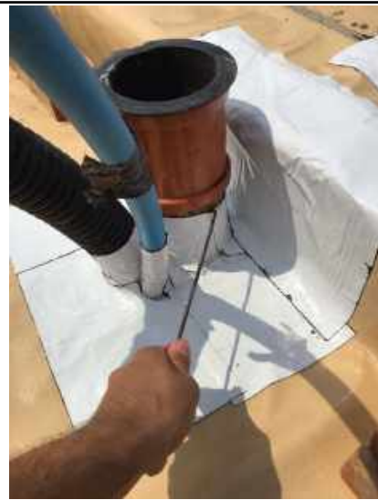
Pick and probe test to a sealed pipe penetration.
