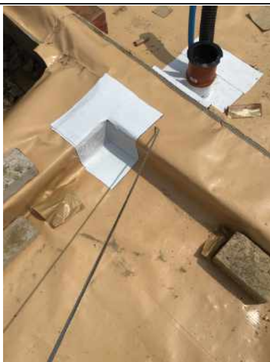
Air lance test to gas resistant self adhesive.
