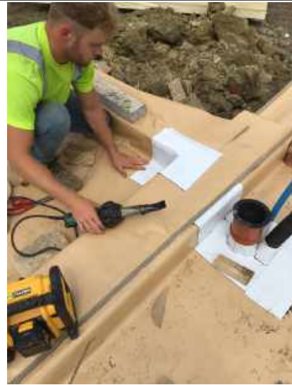
Installer using a hot air leister to seal a corner detail.
