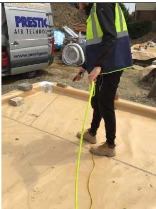
Air lance testing to a welded lap joint.
