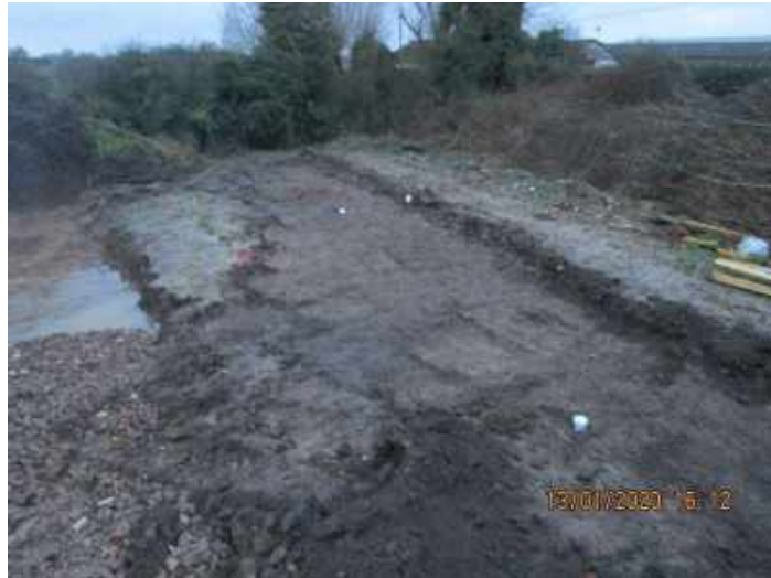
Photo 4 – Extent of remedial excavation and positions of validation samples
