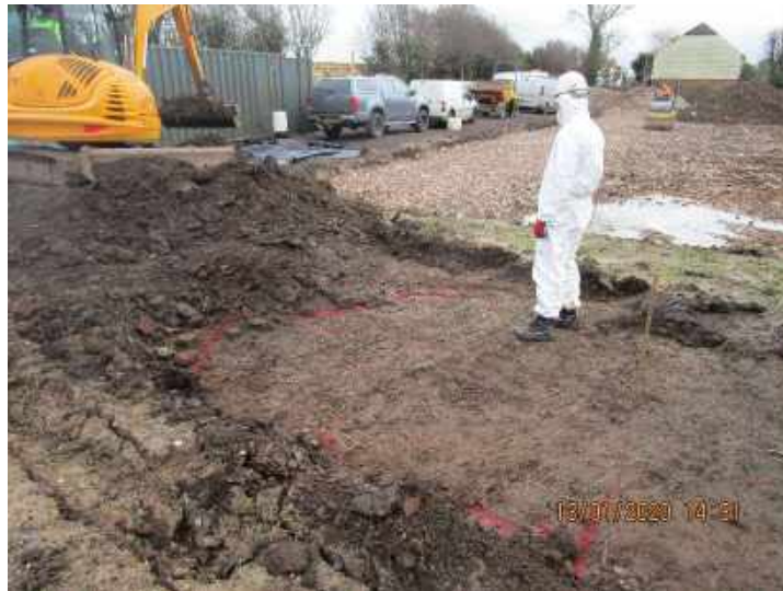
Photo 2 – Contaminated arisings excavated on to plastic sheeting adjacent to the north east of the remedial excavation
