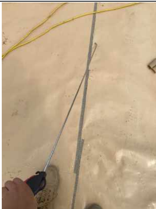
Air lance testing to a welded joint.
