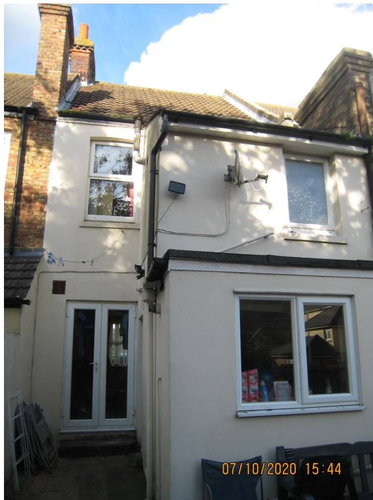
Figure 1 – Existing Back Terrace
