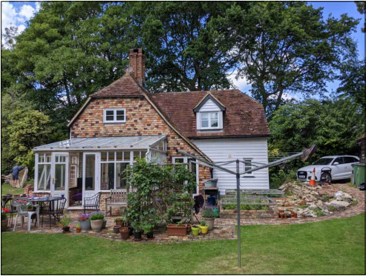
Photo 03 View of south elevation
