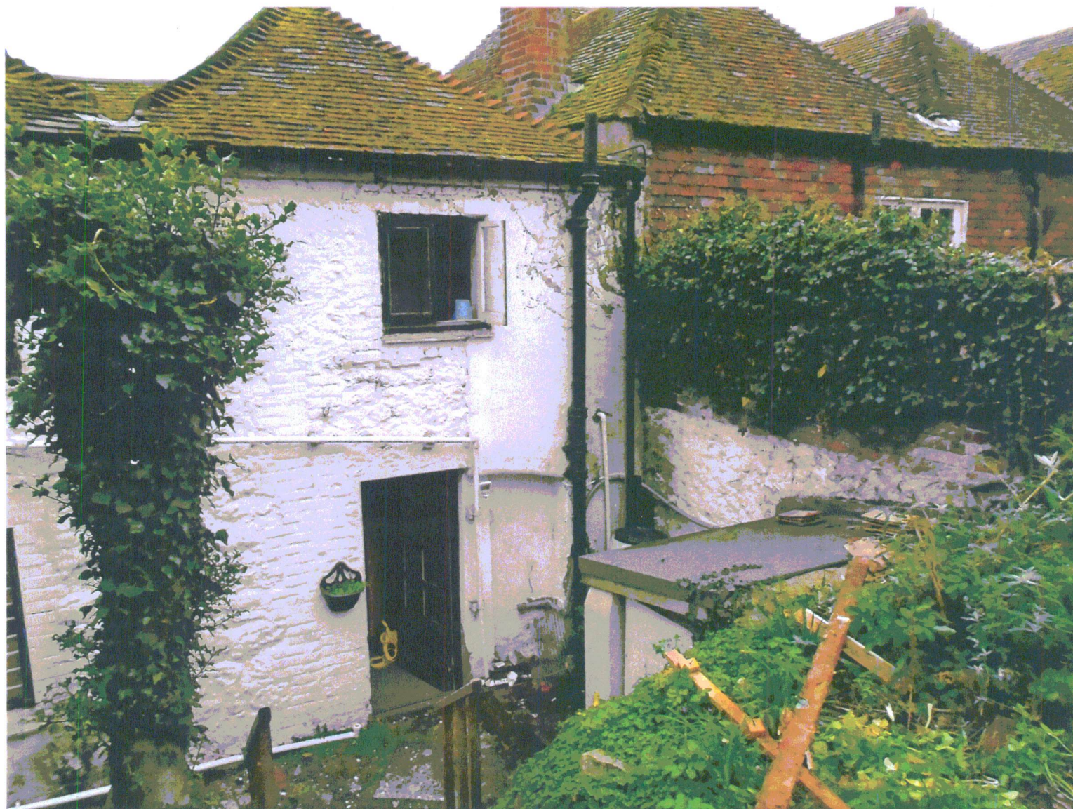
Rear elevation viewed from the garden towards the southwest
