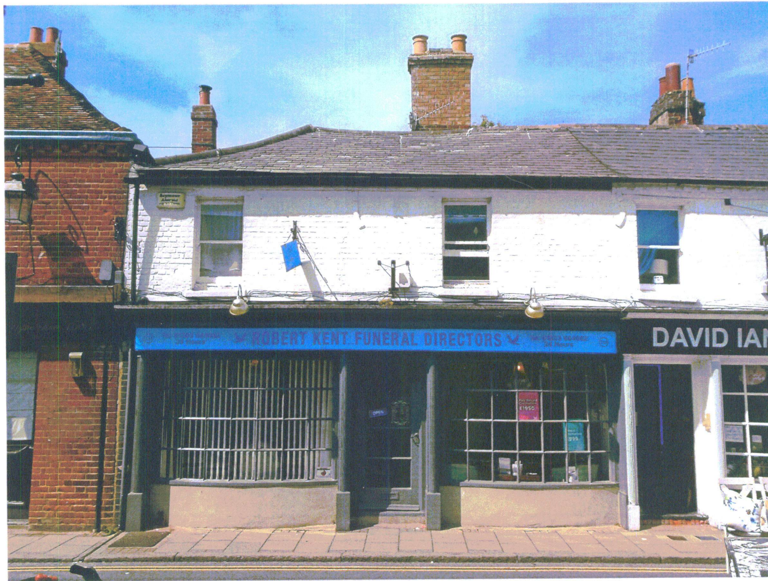
Front elevation viewed from the High Street towards the northwest
