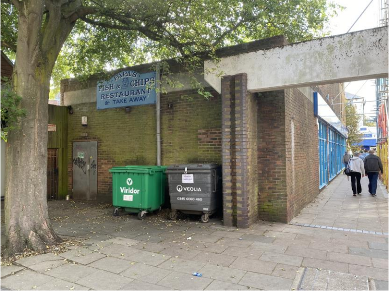
Rear of Site from Town Walk
