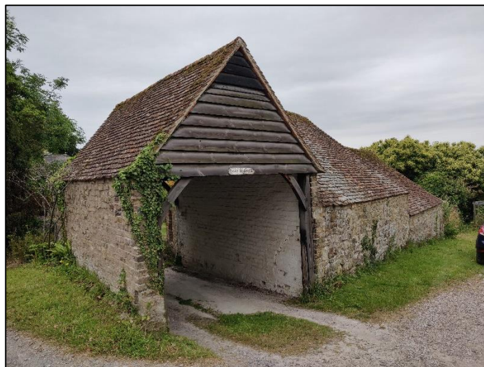
Photo 22: Building B1, double garage building with archway (photo taken 9 th July 2019)
