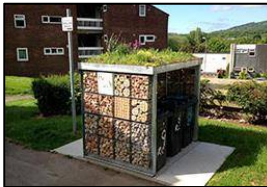
Photo 6.1: Bin store with a green roof and invertebrate houses in the walls (Green Roof Shelters, 2016).
