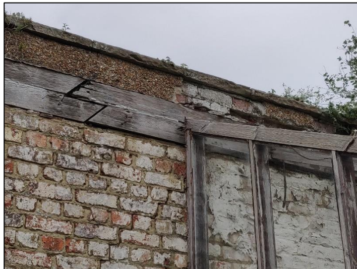
Photo 27: Northern wall structure, situated along the northern border of the site (photo taken 9 th July 2019)
