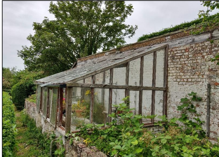
Photo 25: Building B3, greenhouse (photo taken 9 th July 2019)
