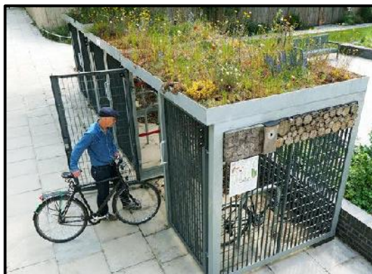
Photo 6.2: Cycle store with a green roof, invertebrate houses and bird boxes installed within the walls (Green Roof Shelters, 2016).
