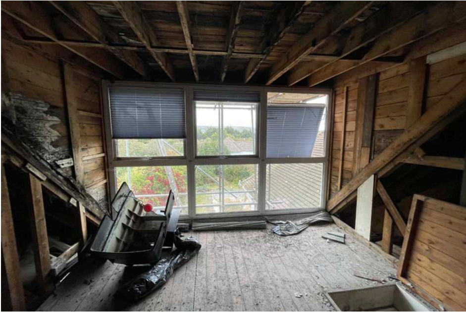
Internal View of Dormer Windows
