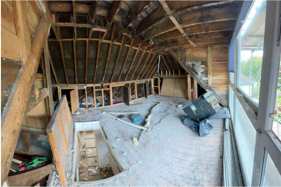
Internal View from Dormer Windows
