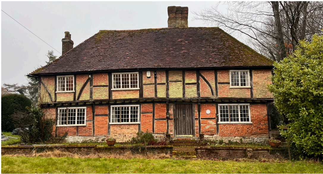
View of main seventeenth-century range of house, looking south (Photo Clague Architects)
