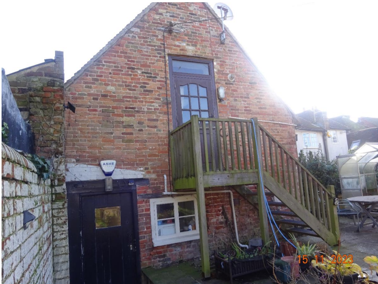
View of rear of building – rendering would be about 800mm high from ground and would run along this wall under window and stairs
