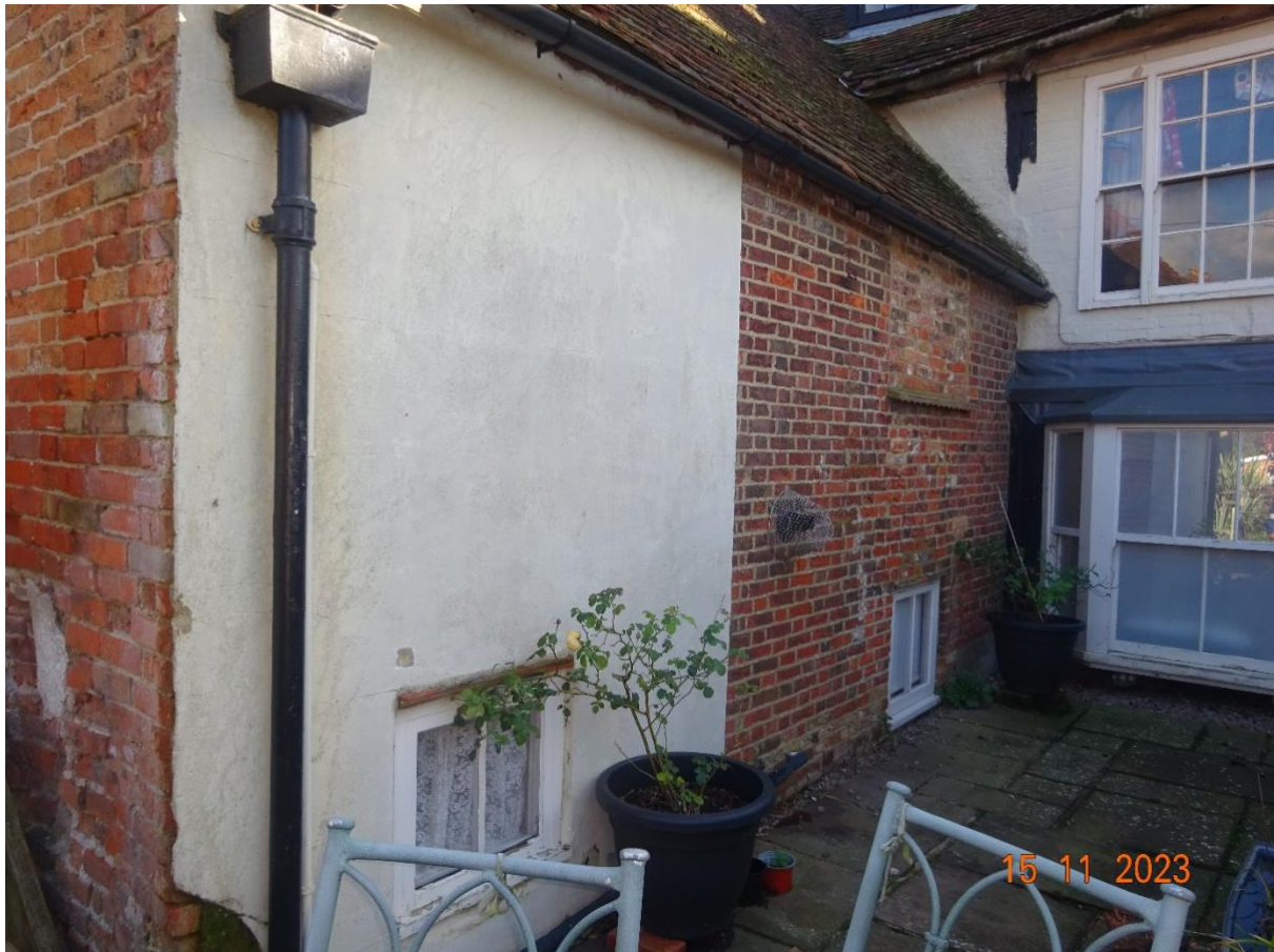
22 High Street side view of rear building, already part rendered.
