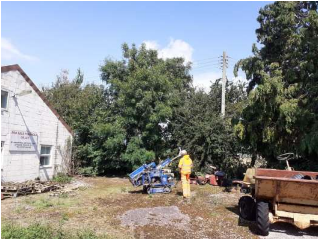
Image of the Windowless Sampler Rig in operation
