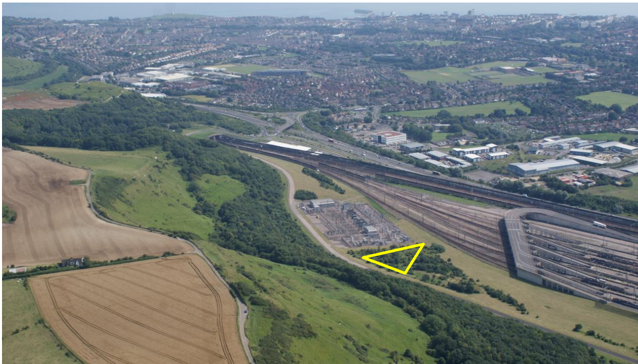
Figure 2.2: Aerial Photograph of the Channel Tunnel portal, at the eastern end of the Eurotunnel UK Terminal at Folkestone, facing south east. The photograph also shows the escarpment in the foreground. The proposed converter station (indicated by the yellow triangle below) would be located adjacent to the existing traction power substation, in the lower right-hand side of the photograph.
