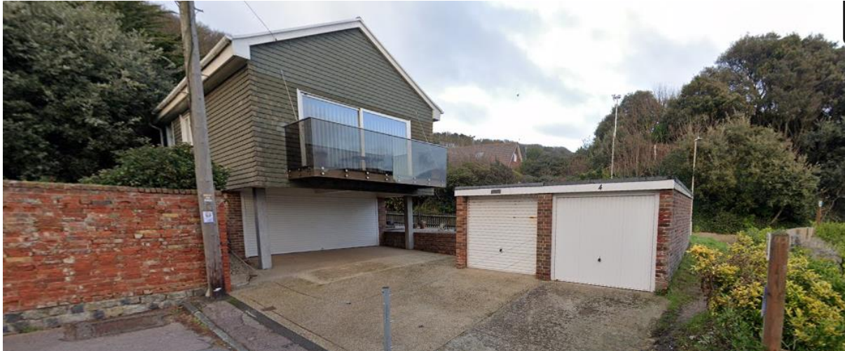
View of the application site from Prospect Road on the eastern edge of the Conservation Area.
