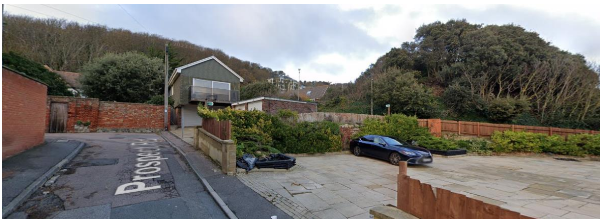
View of the application site from Prospect Road on the eastern edge of the Conservation Area.
