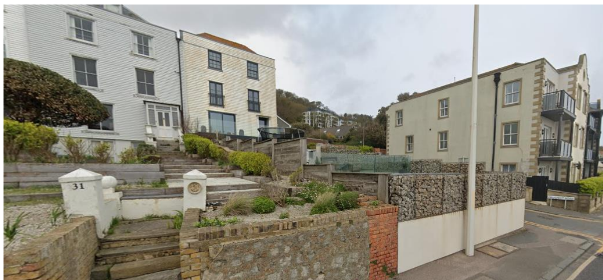
View of the application from Sandgate Esplanade from the eastern edge of the Conservation Area boundary.
