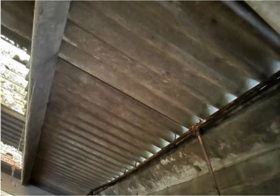
Interior of Roof Barn
