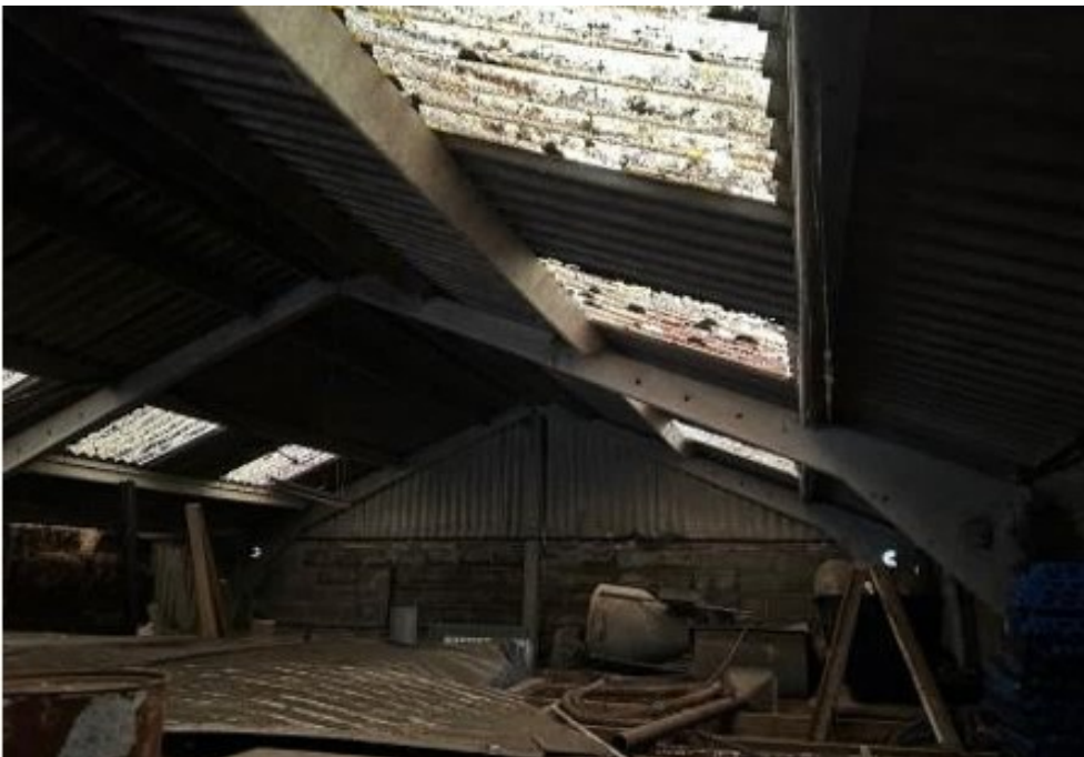
Interior Roof of Barn
