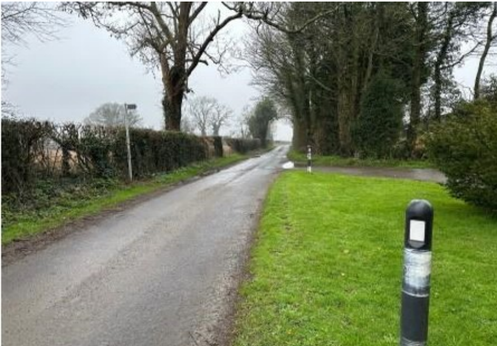
Site Access view westward along Reece Lane.
