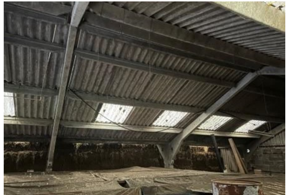
Interior Roof of Barn
