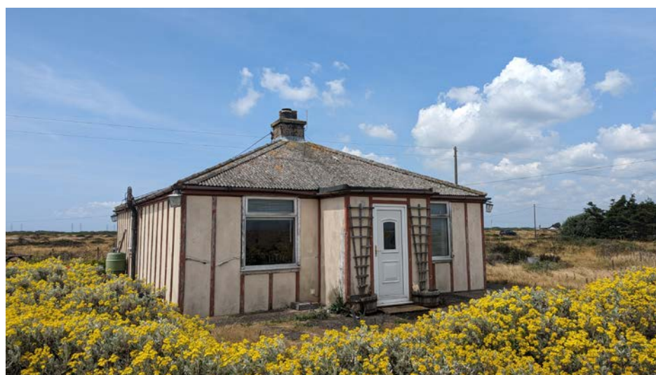
VIEW 04: EAST ELEVATION LOOKING NORTH WEST
