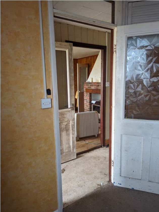
VIEW 06: BEDROOM 01 LOOKING IN TO LOUNGE
