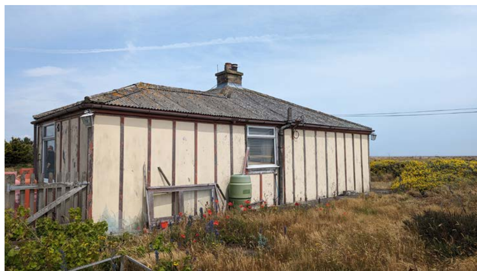
VIEW 05: SOUTH ELEVATION LOOKING NORTH EAST
