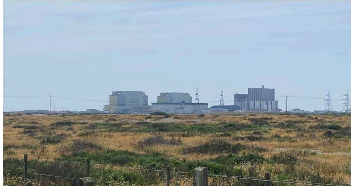
DUNGENESS POWER STATION
