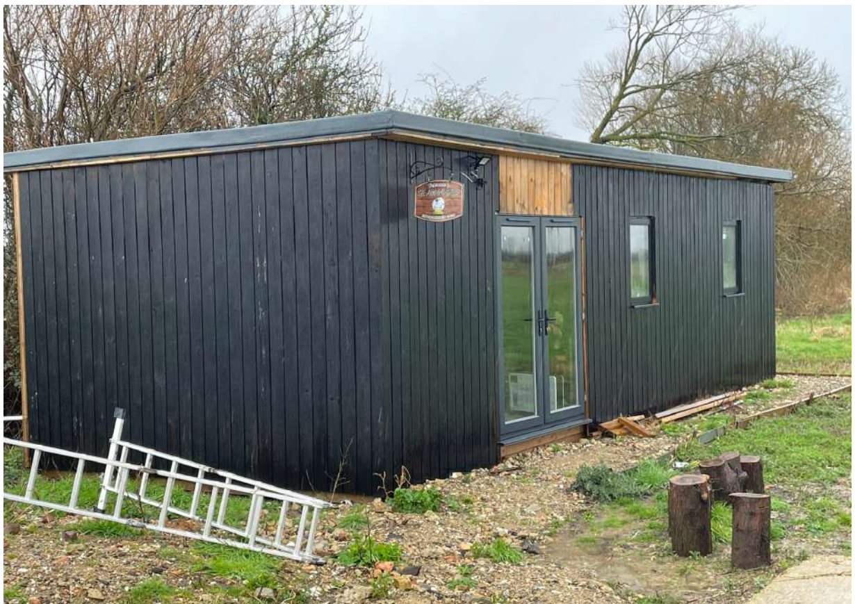
Fig. 10, Photo of the Structure Front Elevation in question (Anske Bax)
