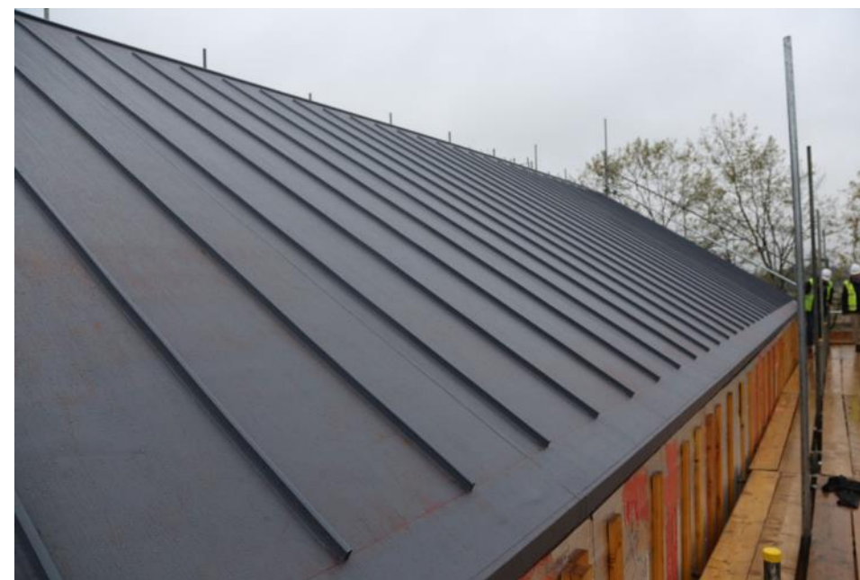
Standing seam type roof covering
