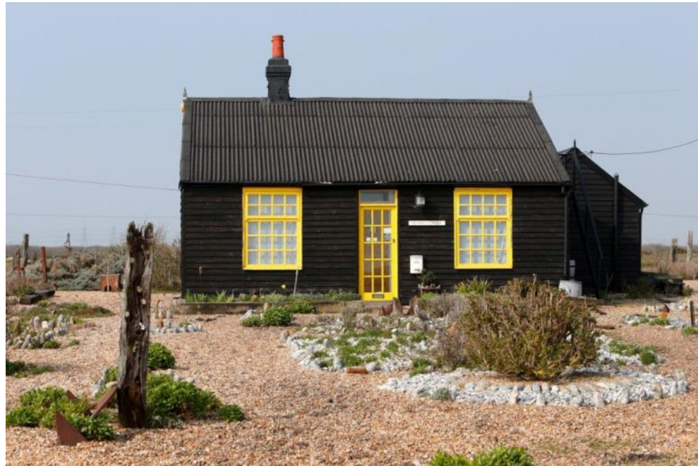
Black cladding New Romney
