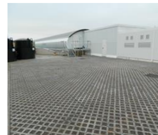
Truckcell heavy duty porous paving
