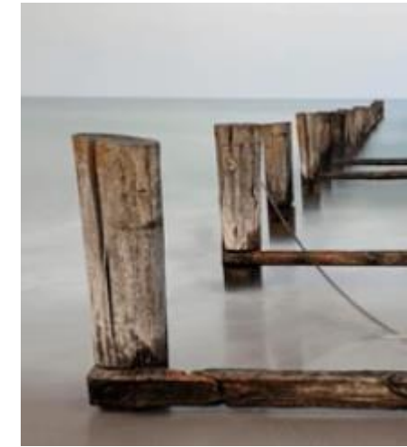
Timber groins—Sea defences
