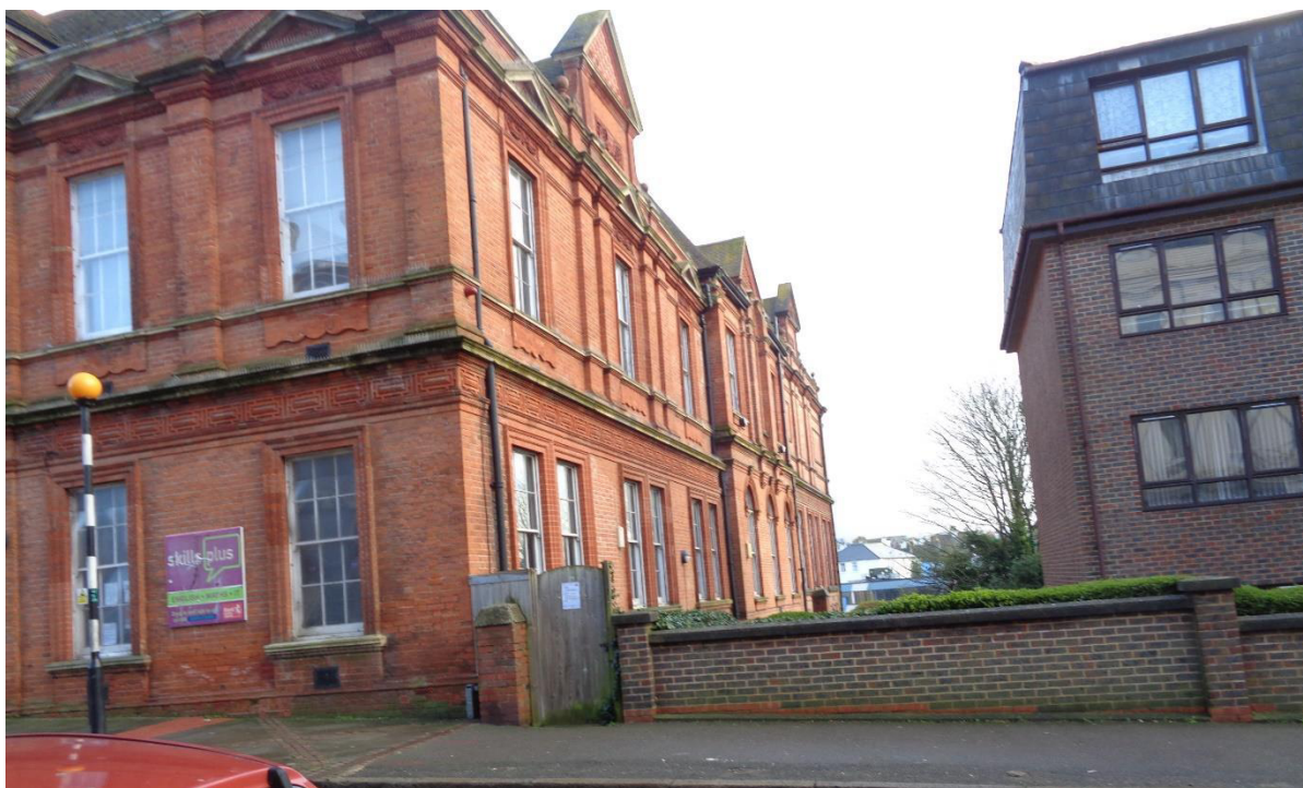
Grace Hill Library Grace Court elevation (Camera 2 & Camera 3)
