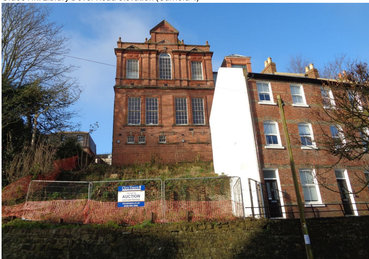
Grace Hill Library Dover Road elevation (Camera 4)
