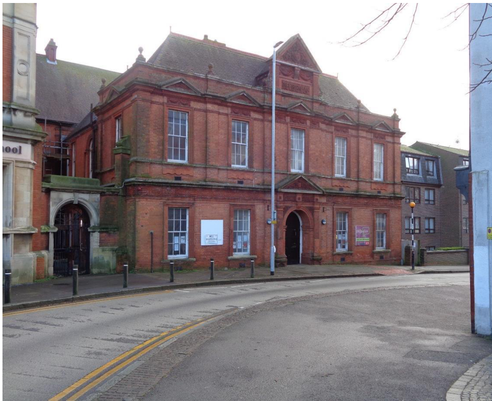
Grace Hill Library Front elevation (Camera 1)
