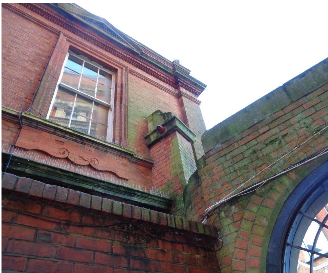
Grace Hill Library Grace Chapel elevation (Camera 6)
