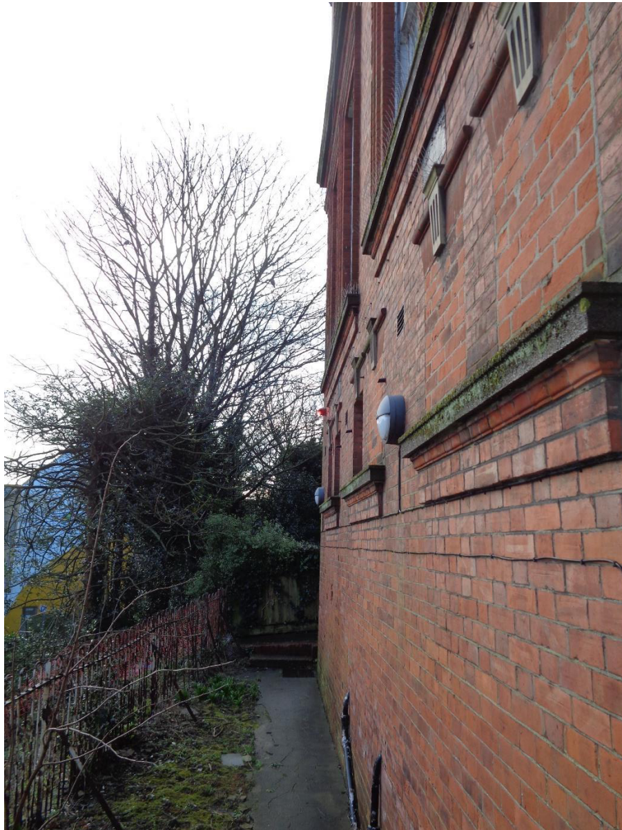
Grace Hill Library Dover Road elevation (Camera 4)
