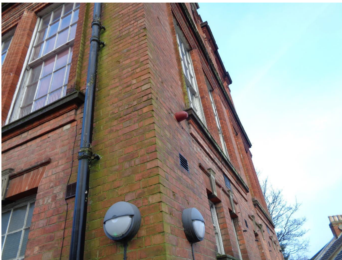
Grace Hill Library Dover Road elevation (Camera 4)
