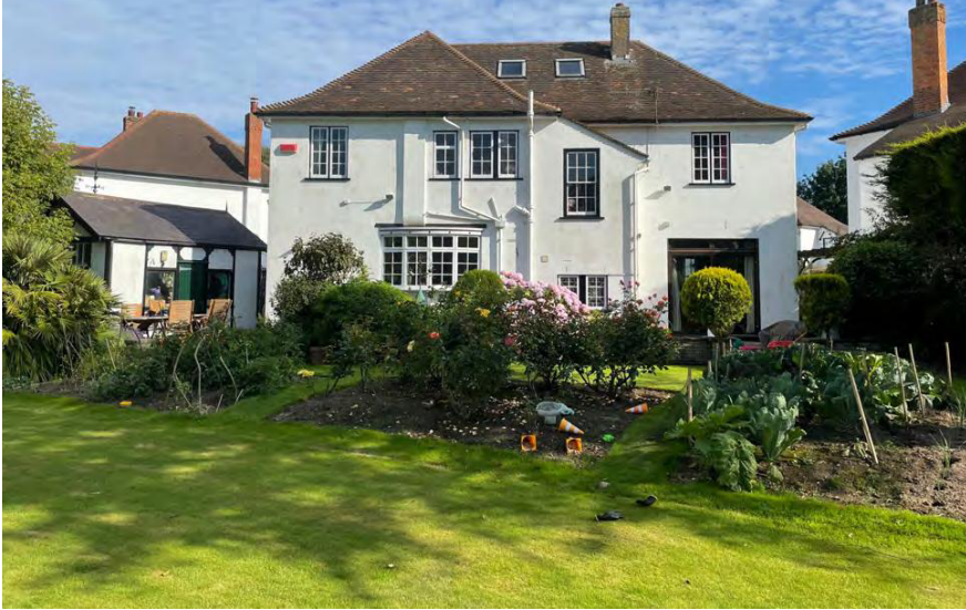
Rear character before works began^
