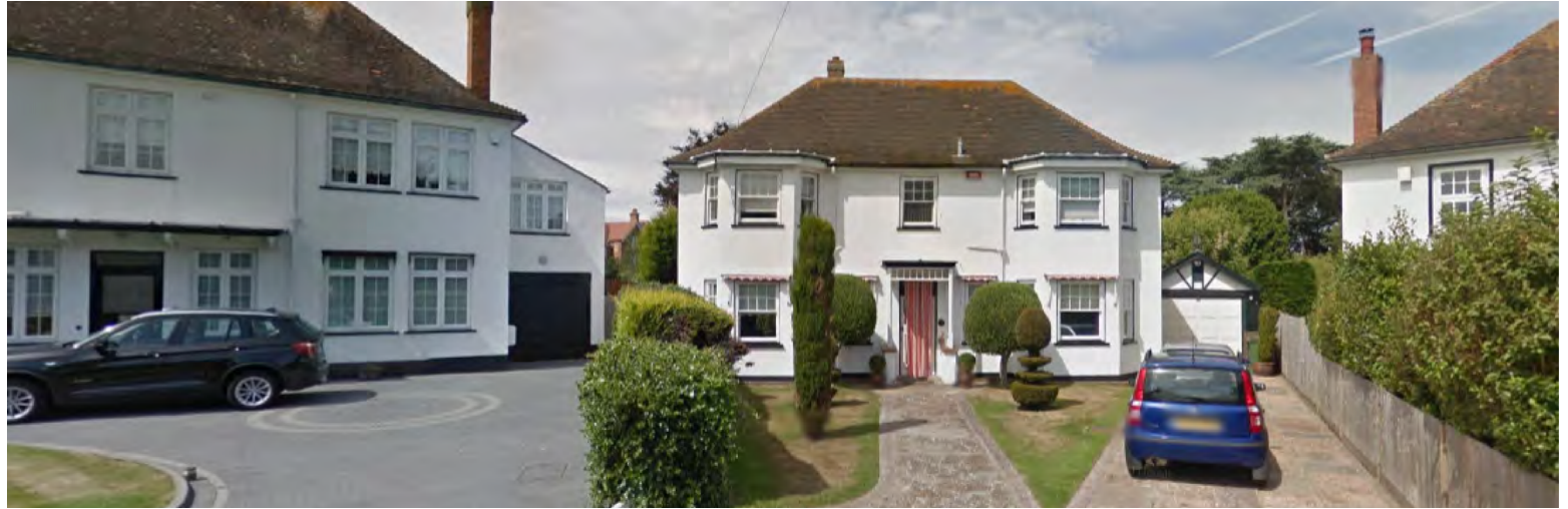
Site before works began ^
