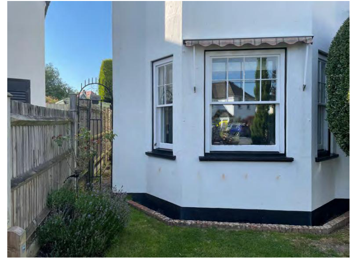
Side access & Window details
