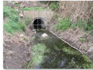
✔ IMG_5689 culvert head of eastern ditch
