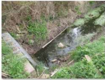
✔ IMG_5687 Eastern ditch
